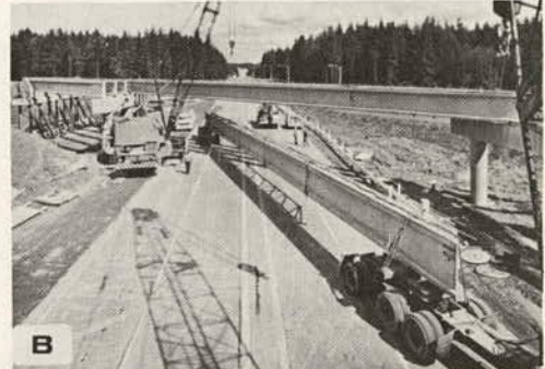
135-ft WS 100 beam delivered by truck and steering trailer (1966)
