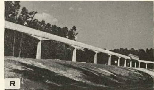
80 percent of expansion joints eliminated by continuity through post-tensioning; smooth guideway ensured by camber and deflection control
