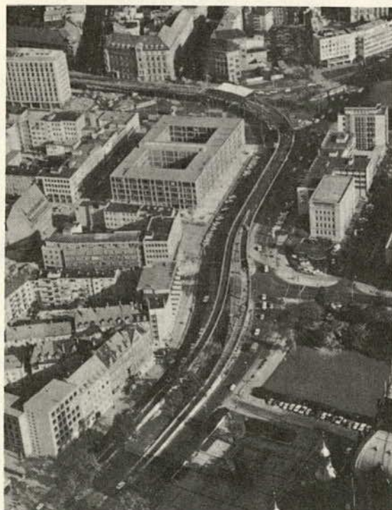
Figure 7. Fast-assembly bridge in Hannover.
