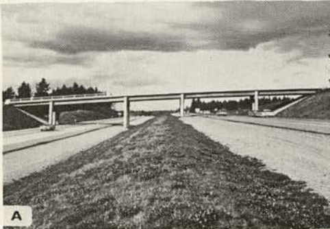
50- to 80-ft simple spans erected in 1960
