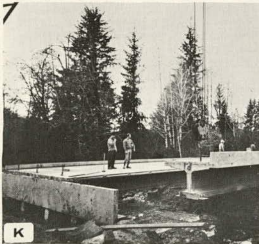
K Girders complete with curbs erected; superstructure placed in 8 hours
