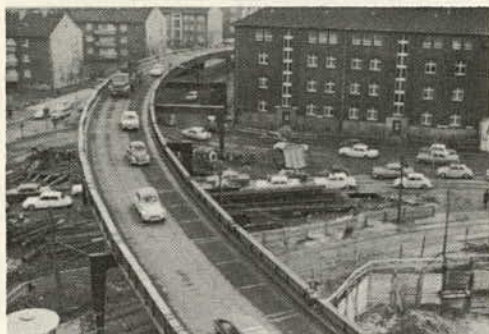
Figure 4. Fast-assembly bridge in Essen where, because of traffic areas underneath, supports are located away from bridge.
