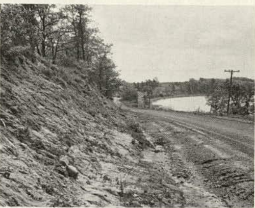
Figure 3. Example of erosion on town road (source: SCS).
