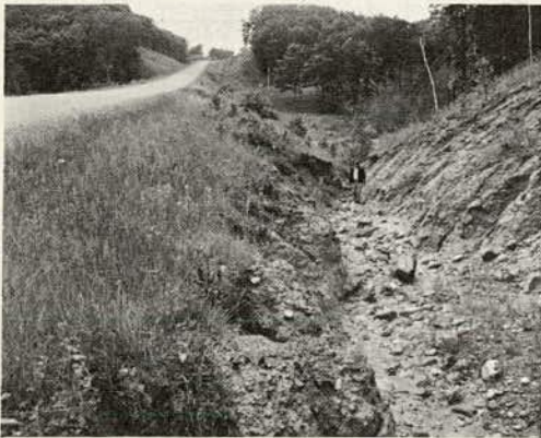
Figure 4. Example of roadside needing structure, sloping, fertilizing, seeding, and mulching.
