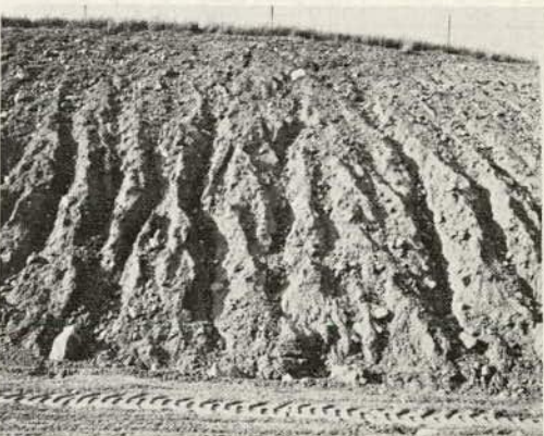
Figure 5. Example of erosion along road under construction.
