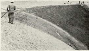
Figure 6. Treatment of excavation with Petroset SB.
