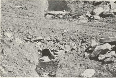
Figure 1. Causeway constructed across stream eliminates need for fording of stream.
