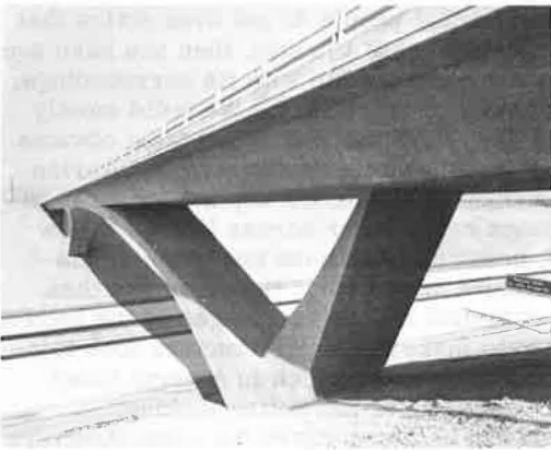
Figure 1. Miramar Road overcrossing near San Diego.
