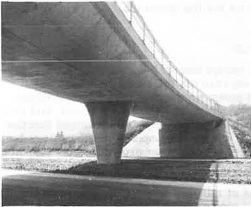
Figure 3. Superstructure with continuous curve from edge to edge.
