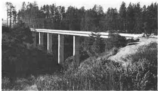
Figure 2. Bridge over Caspar Creek ravine near the ocean.
