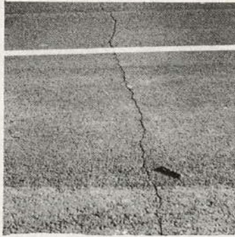
Figure 4. Non-load-associated crack that was thermally induced and may act as catalyst to fatigue cracking.
