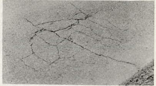
Figure 4. Non-load-associated crack that was thermally induced and may act as catalyst to fatigue cracking.
