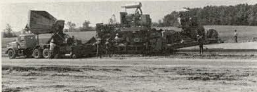
Figure 10. Placement of PCC pavement on CTB.
