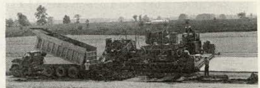
Figure 5. Placement of CTB.
