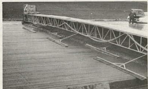
Figure 11. Final finish: longitudinal texturing.
