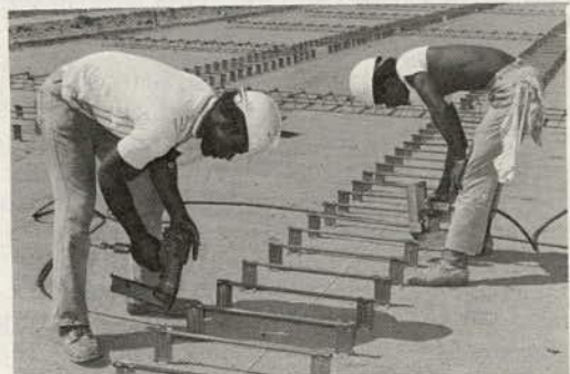
Figure 9. Nailing of supports for tie bars at 1-ft intervals.
