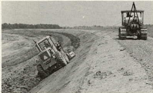
Figure 4. Preparing rough subgrade on curve.
