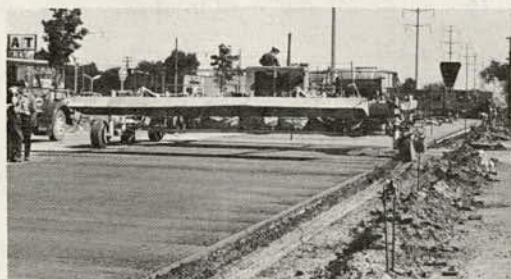
Figure 10. Equipment used to texture and apply curing compound.
