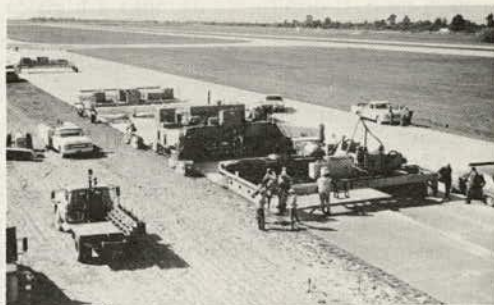
Figure 7. Paving train on 6-in. fibrous overlay.
