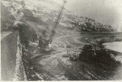
Figure 15. Gabion construction near Glenwood Springs, Colorado.
