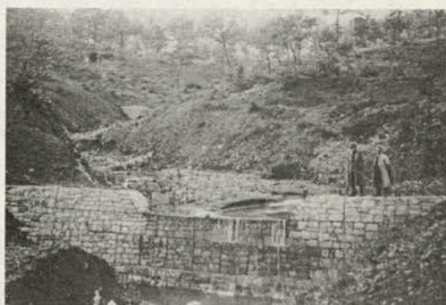
Figure 7. Restoration of a small stream in Europe.
