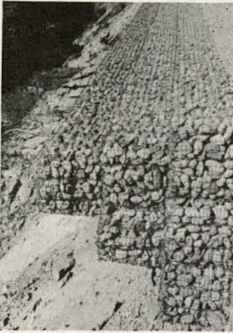
Figure 20. Completed gabions.
