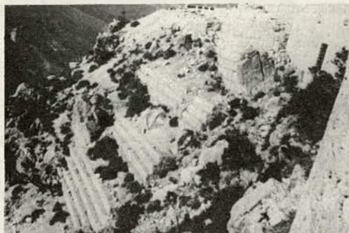
Figure 5. Extensive use in retaining a highway in the Italian Alps.
