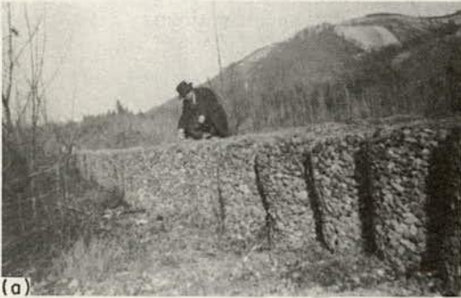
Figure 2. Installations (a) to close a breach in the bank of the River Reno built in 1893 and (b) on the River Santerno.
