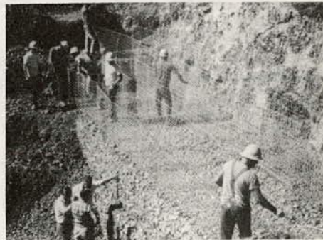
Figure 14. Gabions supporting US-95 near Whitebird, Idaho.
