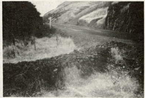
Figure 4. A groin built of stone and hog wire about 1930.
