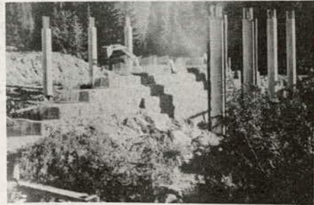
Figure 12. Wall to contain fill at bridge abutment on the Snoqualmie Pass.
