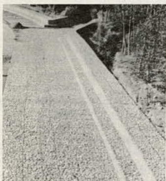
Figure 6. Installation on the River Arno.
