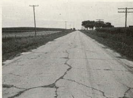
Figure 13. Crack pattern on Greene County project.
