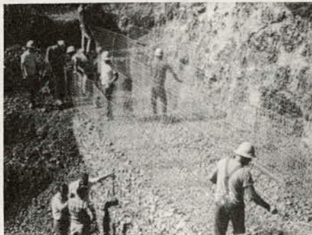
Figure 14. Gabions supporting US-95 near Whitebird, Idaho.
