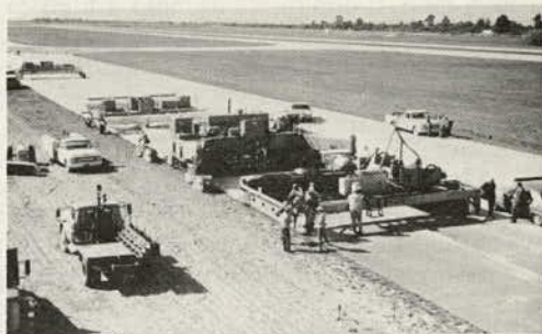
Figure 7. Paving train on 6-in. fibrous overlay.
