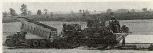
Figure 5. Placement of CTB.
