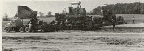
Figure 10. Placement of PCC pavement on CTB.
