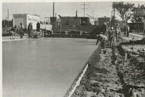
Figure 9. Slip-form paver used on Michigan fibrous overlay.
