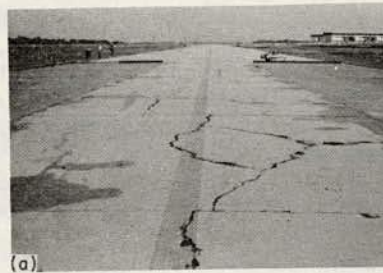
Figure 4. Random (a) longitudinal and (b) transverse cracks in taxiway pavement prior to 6-in. fibrous overlay.
