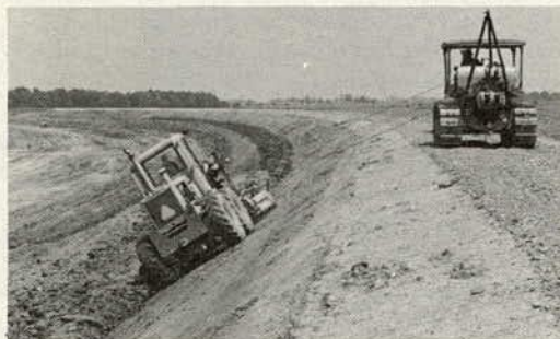
Figure 4. Preparing rough subgrade on curve.
