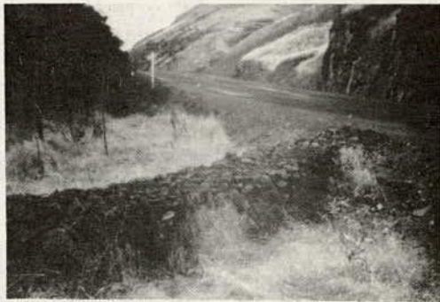
Figure 4. A groin built of stone and hog wire about 1930.
