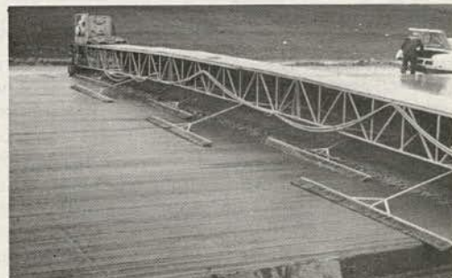
Figure 11. Final finish: longitudinal texturing.
