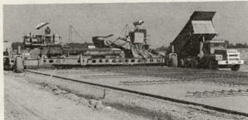
Figure 8. Placement of concrete on west tangent.
