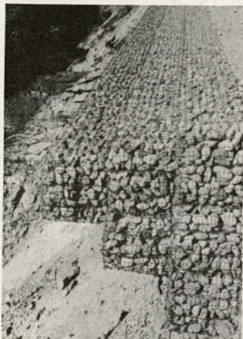
Figure 20. Completed gabions.
