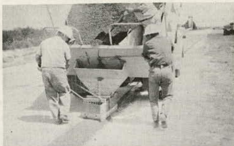
Figure 1. Pavement edge repair.
