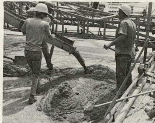
Figure 4. Steel-fiber-reinforced concrete.
