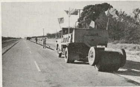
Figure 2. Steel drum roller used to repair pavement edge.
