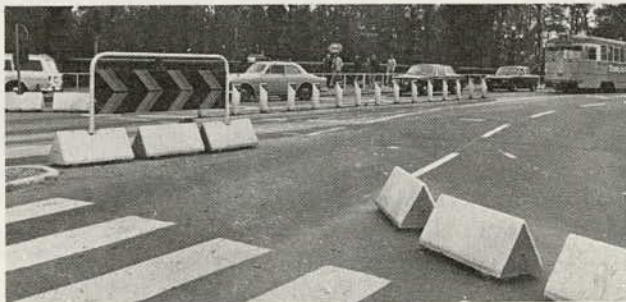
Figure 2. Physical barrier used to direct traffic and outline zone border.
