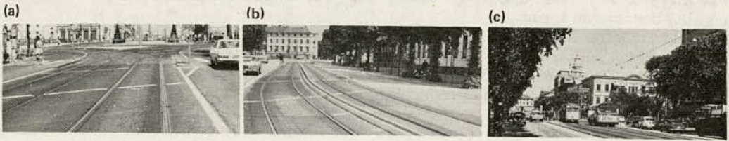
Figure 3. Methods of outlining borders between zones: (a) painted lines, (b) concrete string in middle of border area, and (c) concrete barrier glued to pavement.
