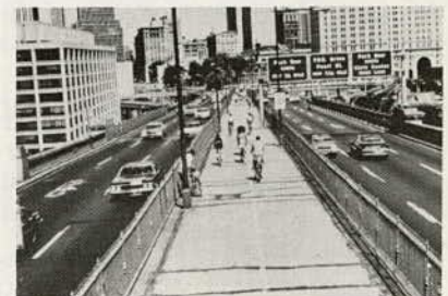
Figure 6. Brooklyn Bridge Bike Path in New York City.
