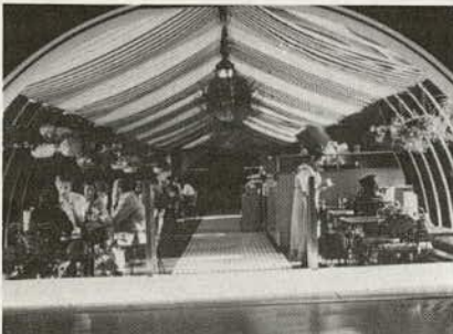
Figure 21. Pedestrian bridge in Denver.
