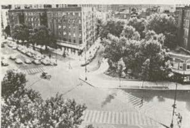
Figure 12. Pedestrian facilities on the Avenue of the Americas in New York City.
