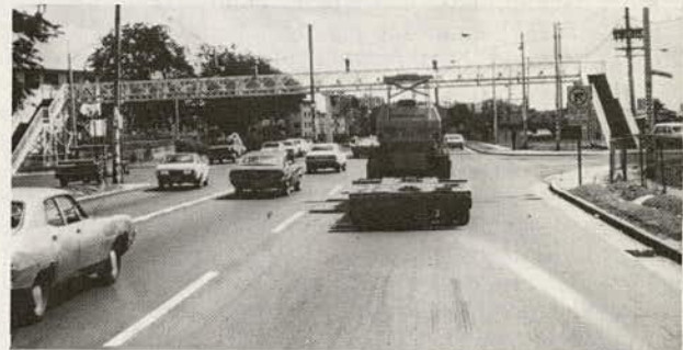
Figure 18. Pedestrian bridge in San Juan.
