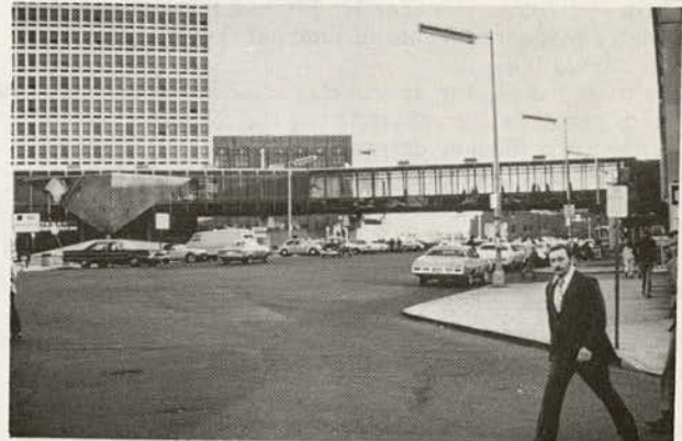
Figure 20. Pedestrian bridge in Newark.
