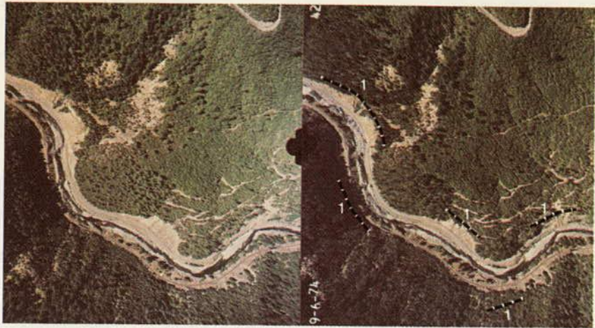
Plate 3.1. Slides in Douglas County, Oregon, caused by undercutting of slopes by stream. Slides largely composed of weathered colluvial materials are evident at almost every bend of stream where it undercuts naturally steep slopes (1). Advantages provided by use of color film include distinction of potentially more unstable colluvial material from more stable bedrock surfaces; ease of distinguishing seepage areas; and indication of vegetation under stress due to insufficient moisture, which could occur because of slope movement.
