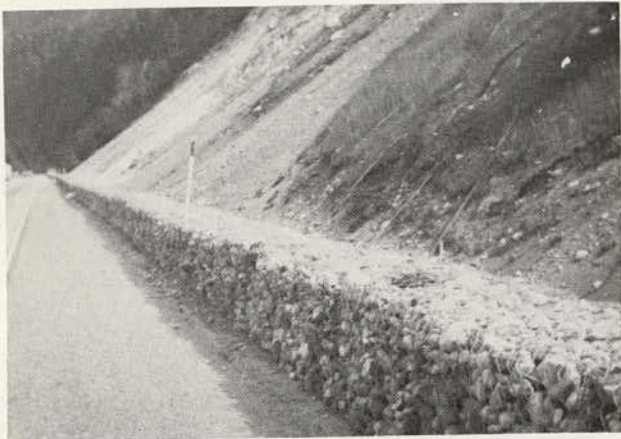
Figure 9.53. Rail and tie wall founded on masonry wall to prevent rolling rock from reaching track of Austrian Railway.
