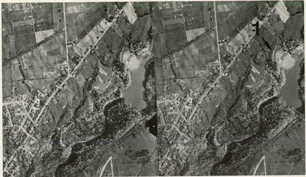
Plate 3.4. Black-and-white photographs taken October 25, 1954, of delta deposits overlying lake bed in Tompkins County, New York. Many landslides in glaciated areas occur in lake-bed materials overlain by granular deposits. Slides occur on both sides of creek. Benching and other slope-stabilizing practices were incorporated to stop sliding. Large landslide is easily identified (1), but evidence of seepage and boundary between delta and lake-bed deposits is subtle and difficult to distinguish on this film type.
