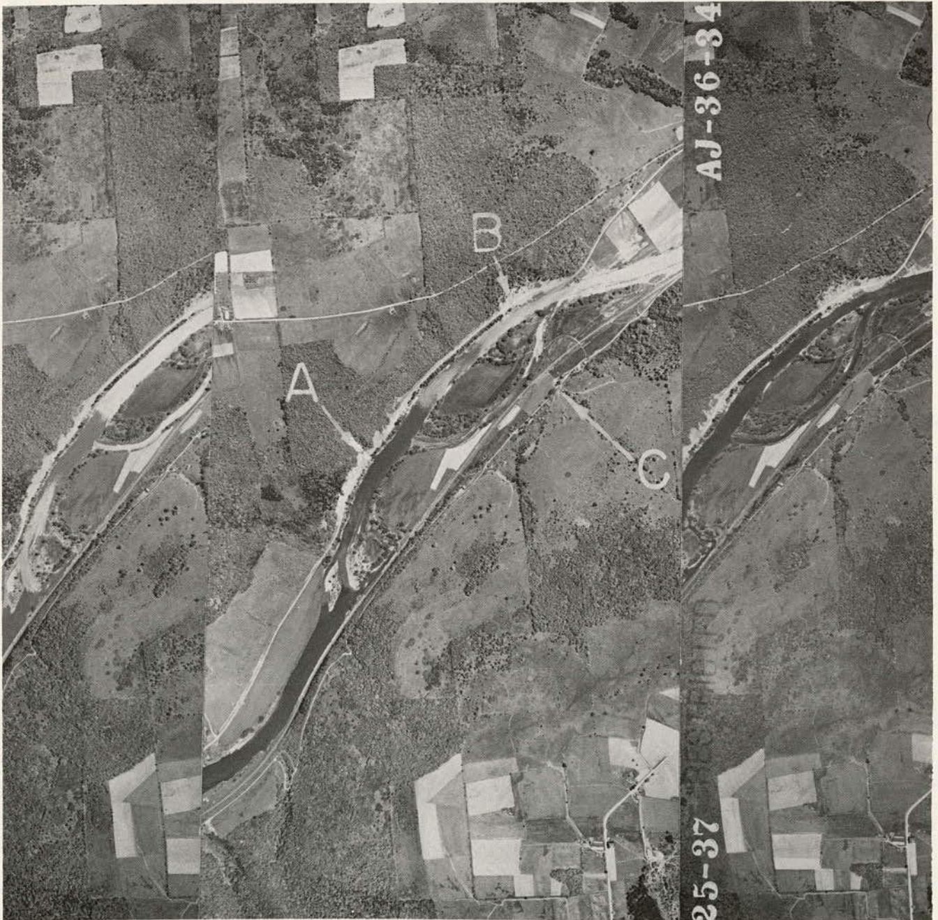
Figure 3.23. Thin till deposit overlying bedrock in glaciated valley in Broome County, New York. Highway cuts in hillsides oversteepened by glaciation create slides (A and B). Slides generally extend to full depth of soil material until competent rock bed (in this case sandstone) is encountered. Between A and B, section of highway entirely in rock has not experienced any slides. In this respect, landslides serve as indicators of depth of soil to rock. On other side of river, site of future slide is indicated at C, an area of concentration of drainage, loose fill, and lack of bedrock control.
