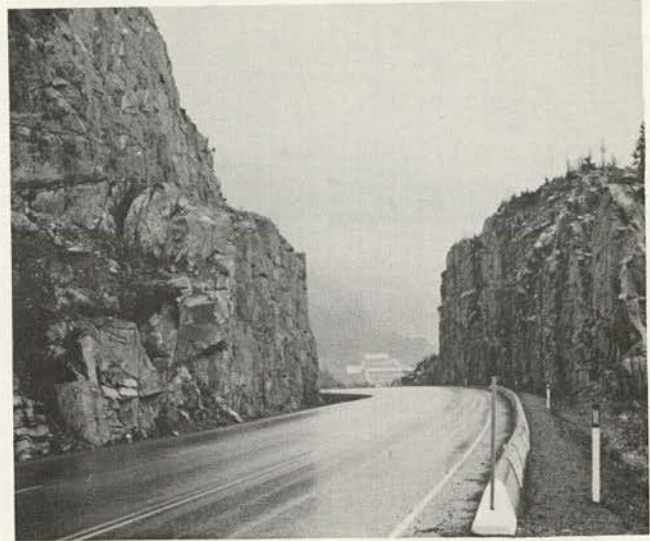
Figure 9.13. Forty-three-meter (140-ft) presheared through cut involving 130 000 m 3 (170 000 yd 3 ) near Britannia, British Columbia, and including cut bench to protect highway from rock falls. Photo is toward south, but sketch is toward north.
