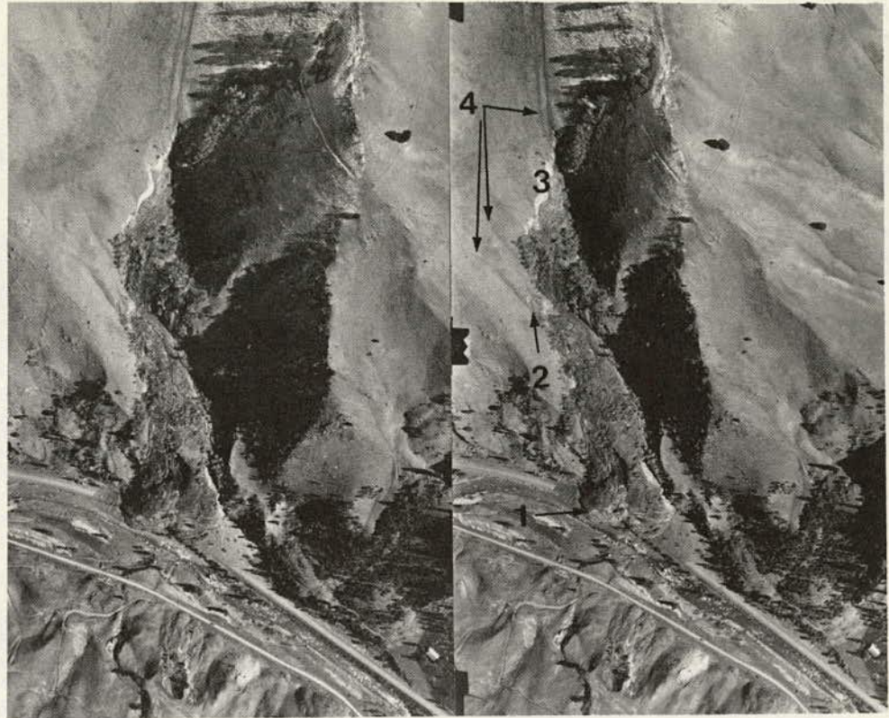
Figure 3.7. Sequential photography for use in evaluation of recent slide development along US-95 in Idaho County, Idaho, and investigation of possible further movements. Aerial photography (top) taken in February 1974 shortly after occurrence of slide (1) shows features present at crown of slide that forewarn of further movement: fissures above scarp face (2), loose colluvial materials on steep slopes at crown (3), and evidence of water feeding into these loose materials (4). Photography obtained 5 months later in July 1974 (bottom) shows that additional slide movement (5) occurred in areas indicated as potentially unstable in photograph above.
