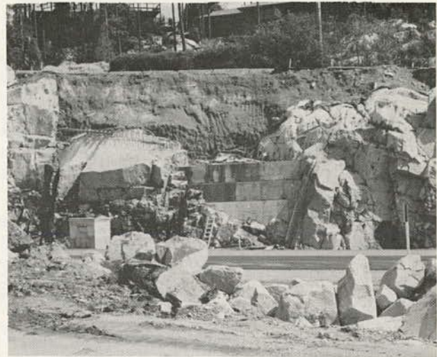
Figure 9.32. Retaining wall (top) that is partly constructed and being cast in place on sound bedrock and finished retaining wall (bottom) with stone facing. In top photo, note broad base of rock dowels that provide for added shear strength at toe of retaining wall as well as excellent bond between concrete and rock.
