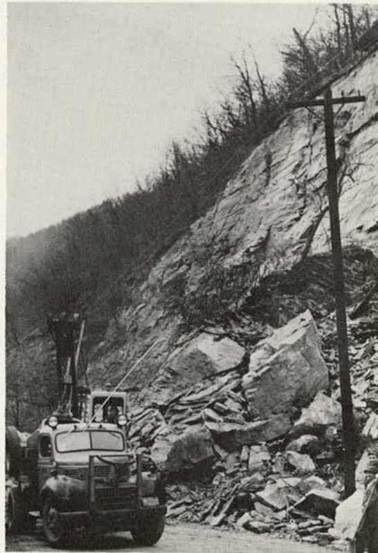
Figure 3.41. Rock slide and rock fall along Penn-105 (3.10). Beds are nearly flat; slide is controlled by joints dipping at steep angle toward road.
