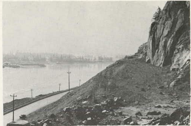
Figure 9.42. Shaped berm that is at toe of high rock face and cut in top of high talus slope above Hope-Agassiz highway in British Columbia.
