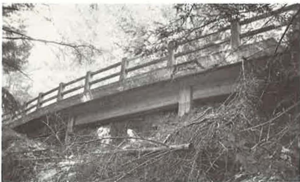
Figure 8.2. Landslide avoidance by bridging near Santa Cruz, California (8.24).
