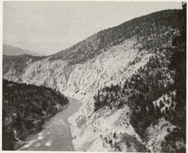
Figure 3.42. Rock fall and rock slide near Skihist, British Columbia, on Canadian National Railroad (3.10). Note bare active slopes, closely spaced jointing of rocks, rock chutes, and absence of water. Wooden and concrete sheds bypass debris falling over tracks from above.
