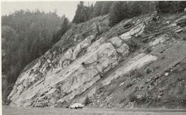
Figure 9.2. Well-developed discontinuities dipping toward highway at Porteau Bluffs, British Columbia. Two significant slides have occurred in this area.
