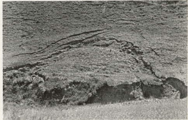
Figure 3.41. Rock slide and rock fall along Penn-105 (3.10). Beds are nearly flat; slide is controlled by joints dipping at steep angle toward road.
