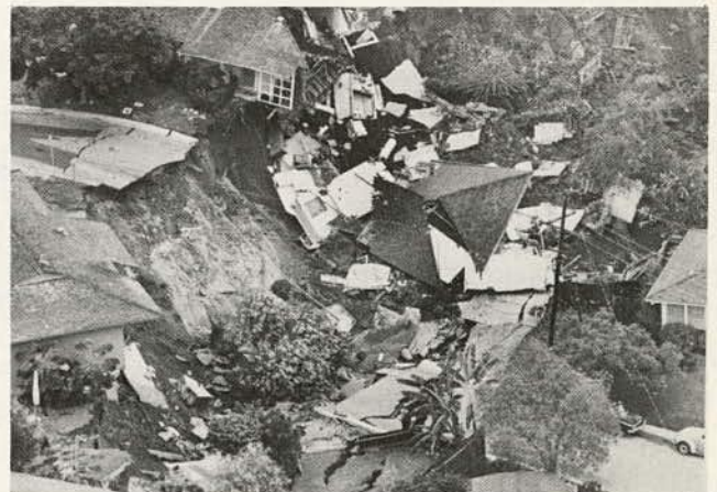
Figure 1.2. Homes and street damaged in October 1978 Laguna Beach, California, landslide.
