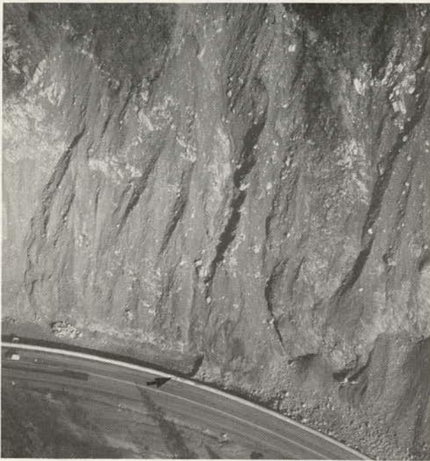
Figure 9.50. Reinforced cast-in-place concrete wall approximately 2 m (7 ft) high and 1 m (3 ft) wide across a major postglacial slide area along edge of Trans-Canada Highway in Fraser Canyon, British Columbia (note break in retaining wall where large blocks have hit wall).
