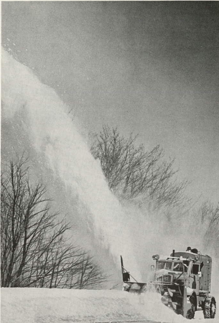
Figure 4. Rotary Plow Dispersing Windrow Formed by V-Plow.
