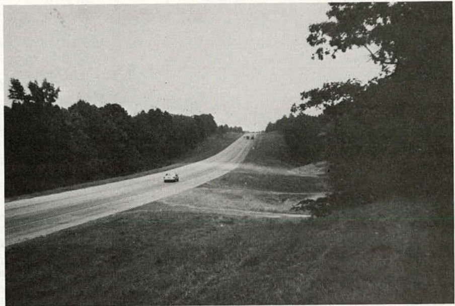
Illustration 8-2. Slow-moving vehicle uses the shoulder of a two-lane rural highway, permitting faster vehicles to pass.
