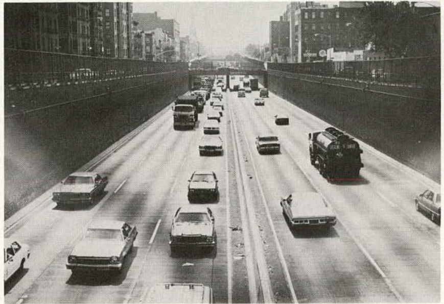
Illustration 3-4. Large gaps in front of trucks or other heavy vehicles are often unavoidable even on relatively level terrain.
