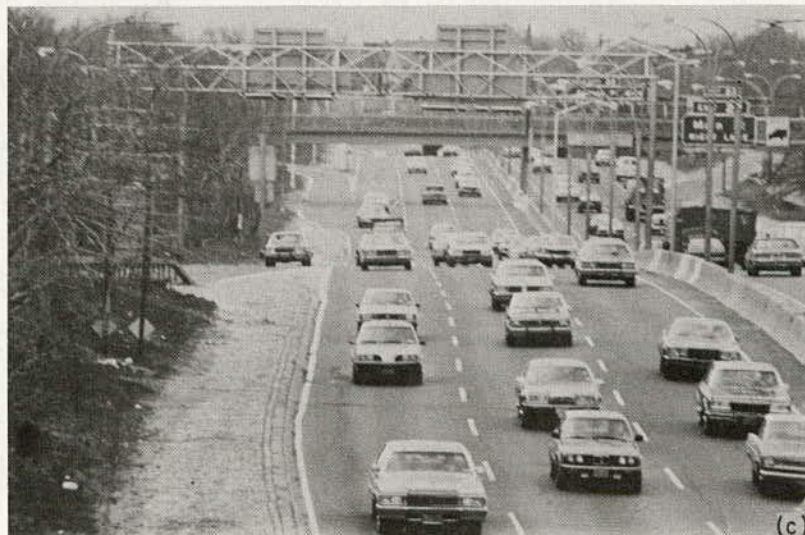
Illustration 5-1. Typical ramp configurations include (a) an isolated on-ramp, (b) an isolated off-ramp, (c) an on-ramp off-ramp sequence.
