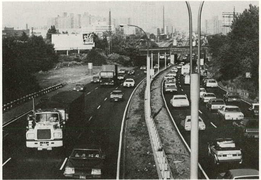
Illustration 3-3. Note formation of large gaps in front of slow-moving trucks climbing up-grade.
