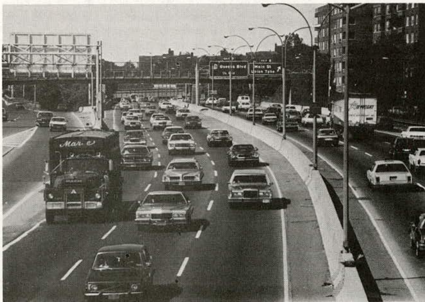
Illustration 3-2. In this case, vehicles shy away from the roadside barrier. This causes a shift towards the median in the placement of vehicles in each lane. This is also an indication that the median barrier illustrated here does not present an obstruction to drivers.
