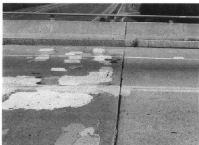
FIGURE 3-5 Patching of a severely contaminated concrete deck.
