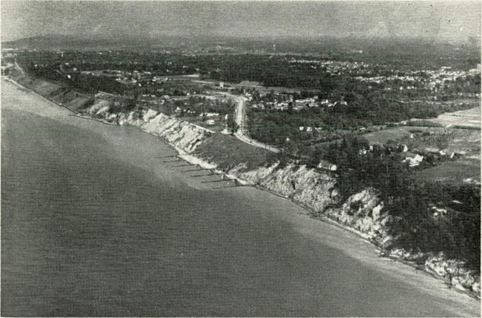
Figure 4. Shoreline erosion on Lake Michigan, U. S. Highway 12, south of St. Joseph, Mich. Shoreline property is valuable; the soilfalls shown here, caused by toe erosion during high lake levels, destroyed costly homes and threatened a major highway. Temporary (?) correction shown consists of slope-flattening, protective sand blanket on slope, and construction of groins to build up beach sand deposits at toe. (Photograph courtesy of Michigan State Highway Department)
