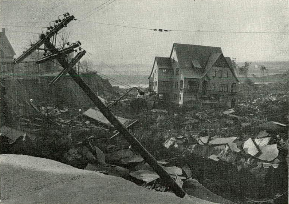
Figure 3. Public and private property destruction on a large scale at Nicolet, Quebec. This slide, a failure by lateral spreading in "sensitive" marine clays, took place without warning on November 6, 1955. It cost a $2,000,000 loss in property and took three lives. The house shown was once at the level of the unbroken ground above it. Except for the greater destruction caused by this one, it is similar to many former slides along much of the St. Lawrence valley. (Photograph by Montreal Gazette)
