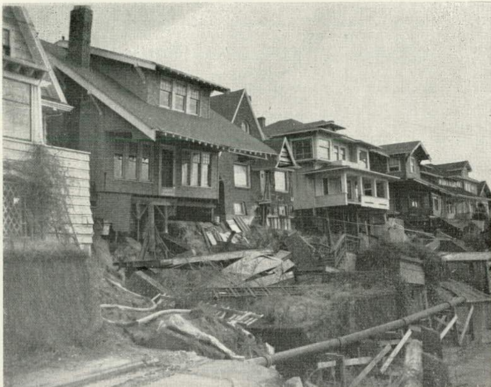
Figure 2. Landslides in cities can wipe out property values. This slump-debris flow in Seattle, Wash., began in 1951 and was still moving in 1956. In lake-deposited silts and clays, it was caused primarily by heavy rains, but overloading of a too-steep slope whose toe had been removed by man and nature was a contributing factor. The street in foreground is demolished and the houses useless; total loss of property value is more than $100,000. (Photograph by D. R. Mullineaux, U. S. Geological Survey)
