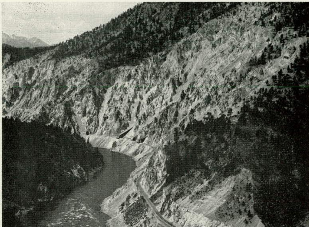
Figure 42. Rockfall and rockslide near Skihist, British Columbia, on Canadian National Railroad. Note the bare active slopes, the closely spaced jointing of the rocks, the rock chutes, and the absence of water. This picture also shows one method of protection against landslides—falling debris from above is bypassed over the tracks by means of wooden and concrete sheds. (Photograph by F. O. Jones, U. S. Geological Survey)
