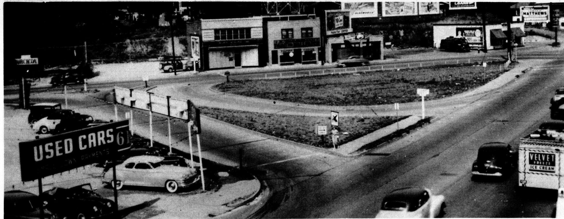
Figure 1. Channelization of intersection of Jennings Station Road, Kienlen Avenue, and Natural Bridge Road, St. Louis County, Missouri. This channelization is designed to eliminate left turns within the intersection.
