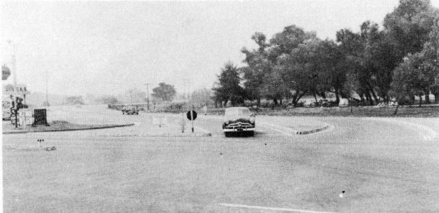
Figure 3. Channelizing islands with reflect-ing curbs.
