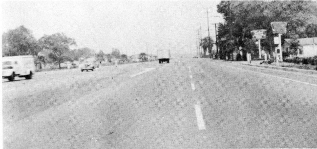
Figure 4. Separated left turn lane on Colton Avenue.
