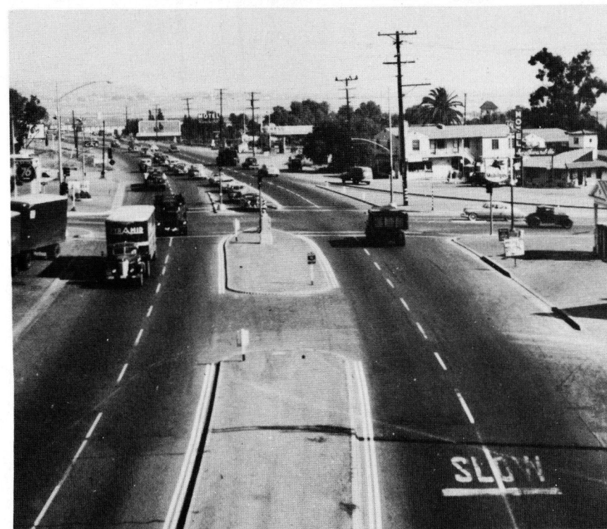
Figure 3. Double line next to reflecting curb improves visibility of median curbs.
