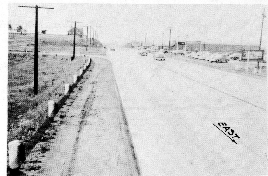
Figure 3. Narrow median on US 40 designed to prevent improper turn into separated right-turn lane.
