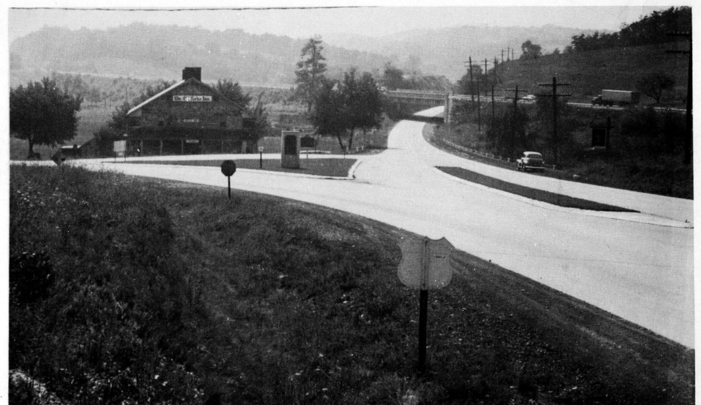
Figure 2. Sloping curbs around islands painted with white reflectorized paint to improve contrast and night visibility.
