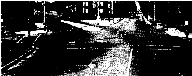
Figure 2. Intersection after channelization. Note that the pedestrian crosswalk has been cut through the median on Pennsylvania Avenue.
