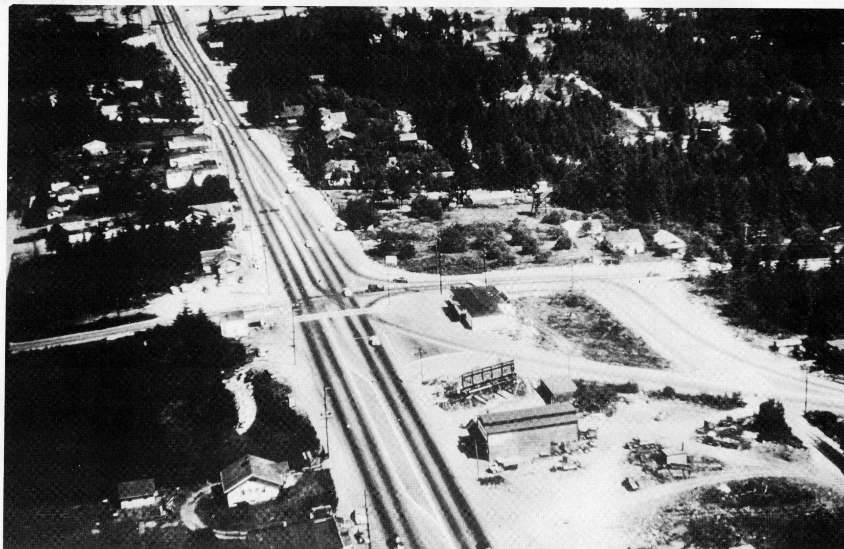
Figure 1. Effective channelization treatment to correct a dangerous intersection: US 99, North 145th Street, and SSH 1-J, near Seattle.
