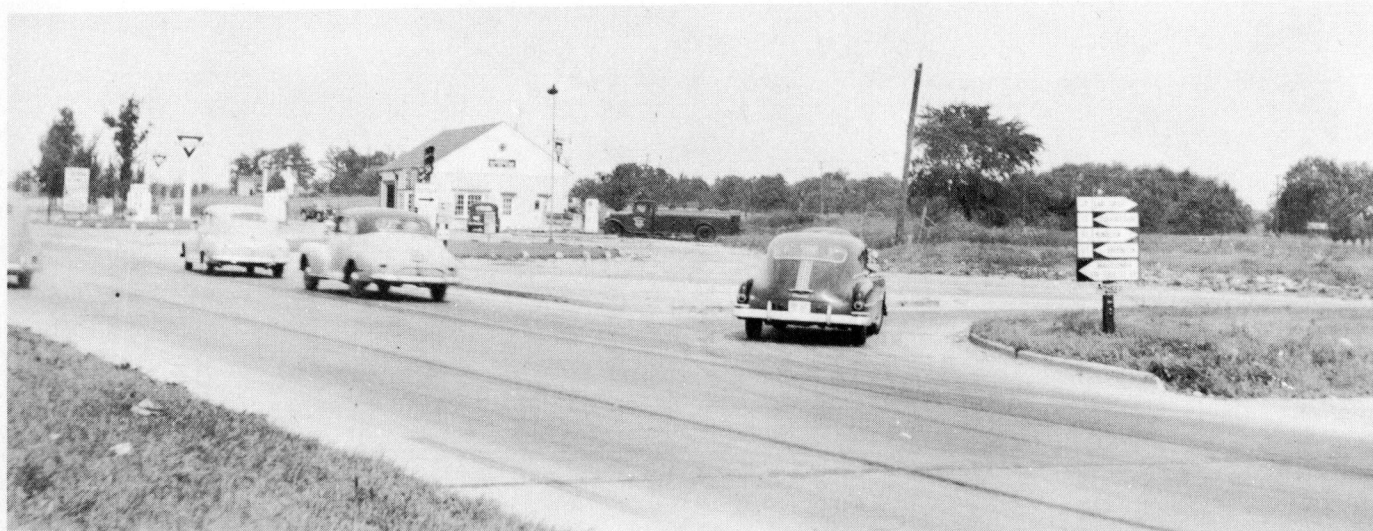
Figure 1. Channelization of acute-angle intersection of high-speed state route, US 12, and secondary highway, Illinois 12 and 22, near Lake Zurich. Right-turn islands provide better placement of signals and remove right turns from intersection.
