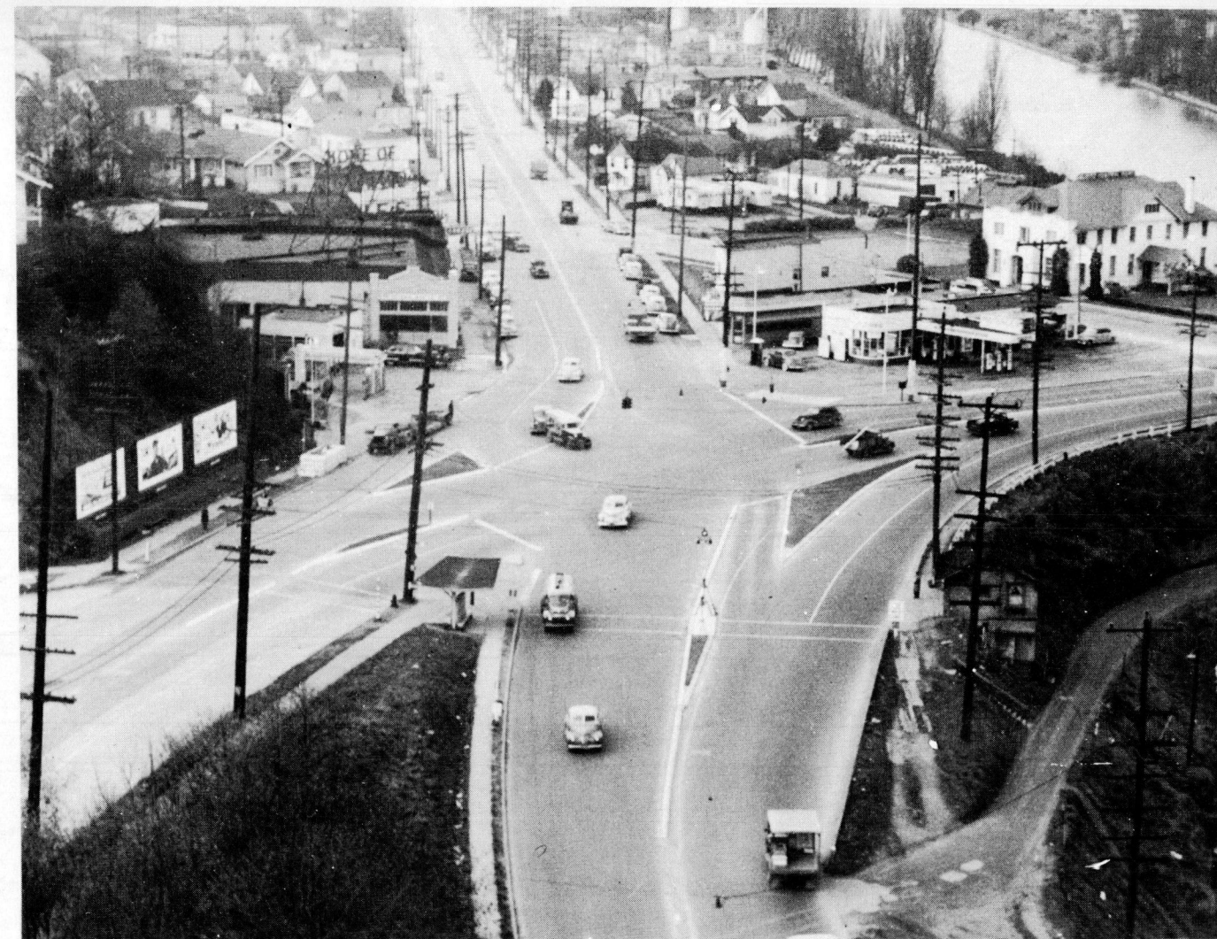
Figure 2. Intersection looking west after completion of channelizing islands and signal controls.
