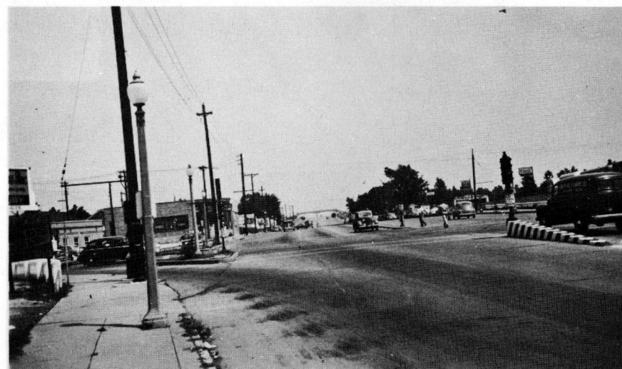
Figure 2. Channelization of Goodfellow Boulevard and Natural Bridge Road, St. Louis.
