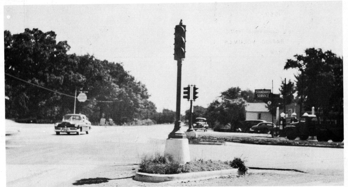
Figure 2. Channelizing island at southwest corner of intersection. Note that the maintenance of planting on small channelizing islands is not practical.
