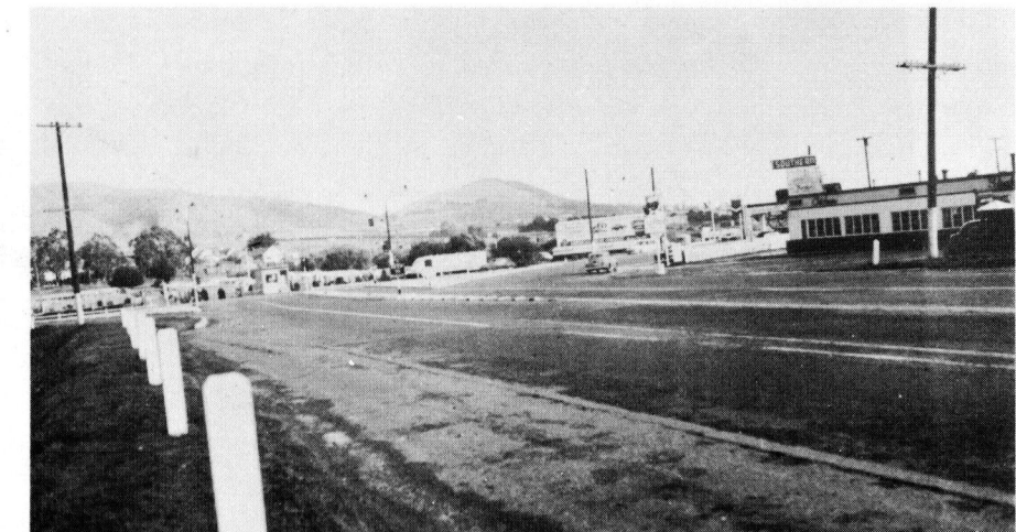
Figure 3. Approach end treatment of divisional island on Junipero Serra Boulevard.
