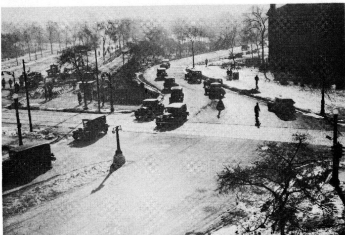
Figure 1. Intersection of 51st Street and South Parkway, Chicago, in January 1936 before channelization, showing dangerous reverse curb on South Parkway, with Washington Park at extreme left. Note the several ancient features.
