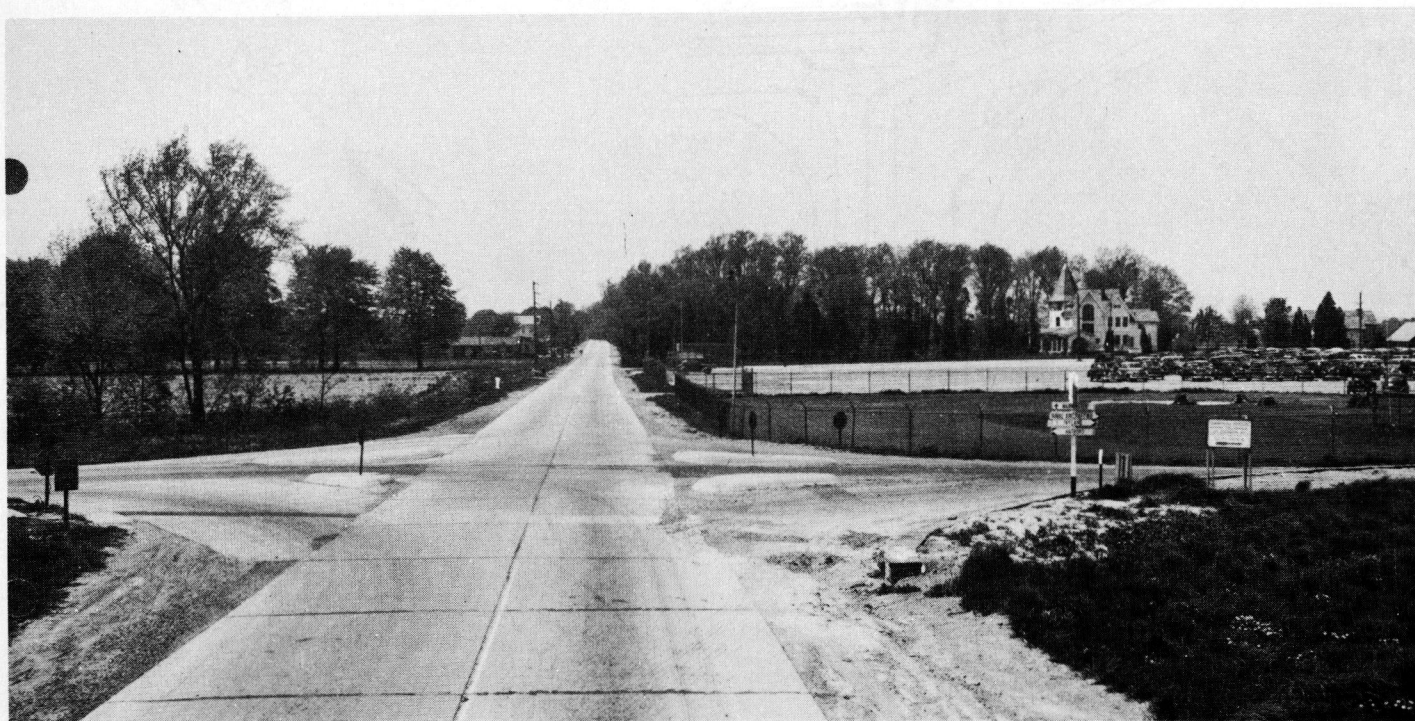
Figure 1. Channelized intersection of Street Road and Jacksonville Road, Bucks County, Pennsylvania. Channelization does not control left turns. Right-turn movements are restricted by short radii and narrow channel widths.
