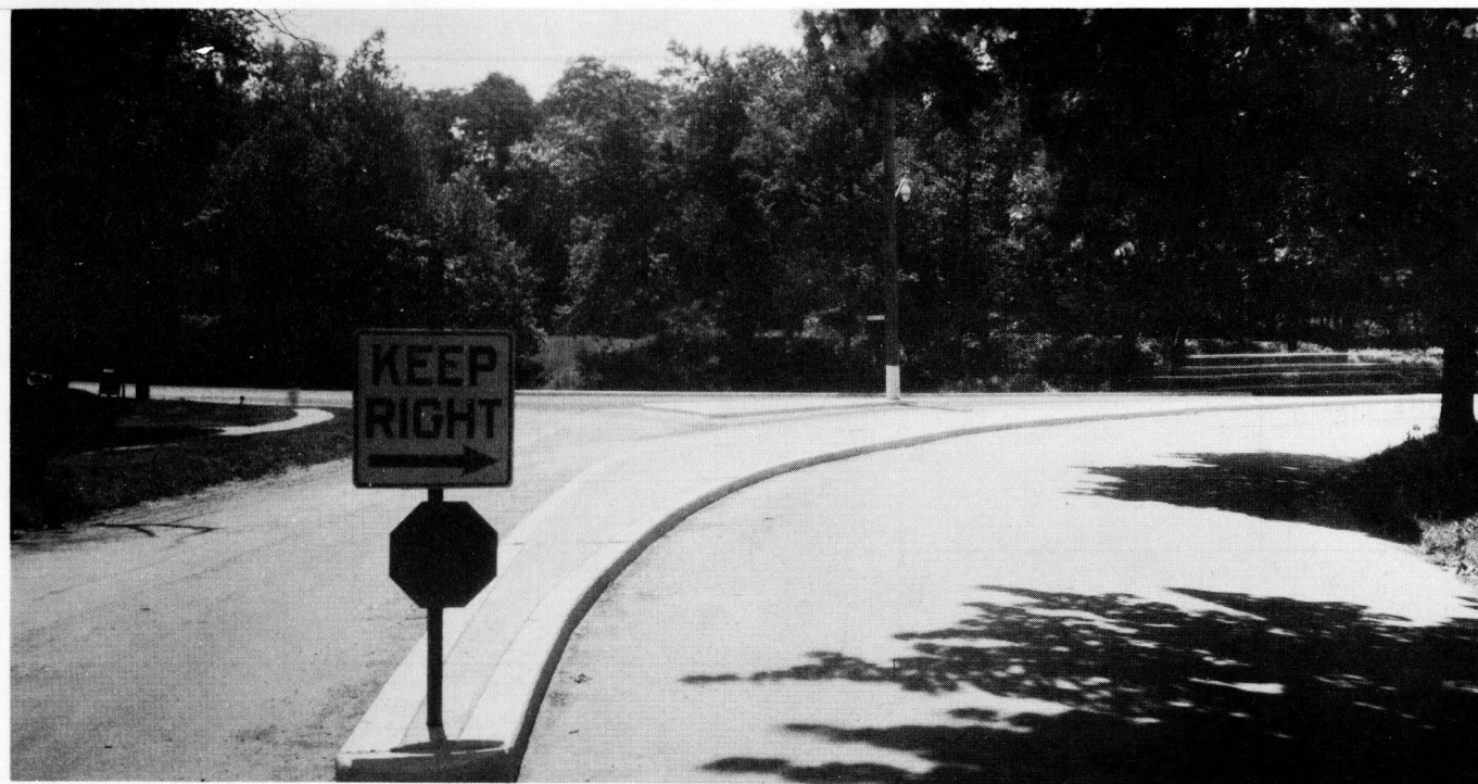
Figure 3. Channelizing island with traffic-control signs on Bryn Mawr Avenue.
