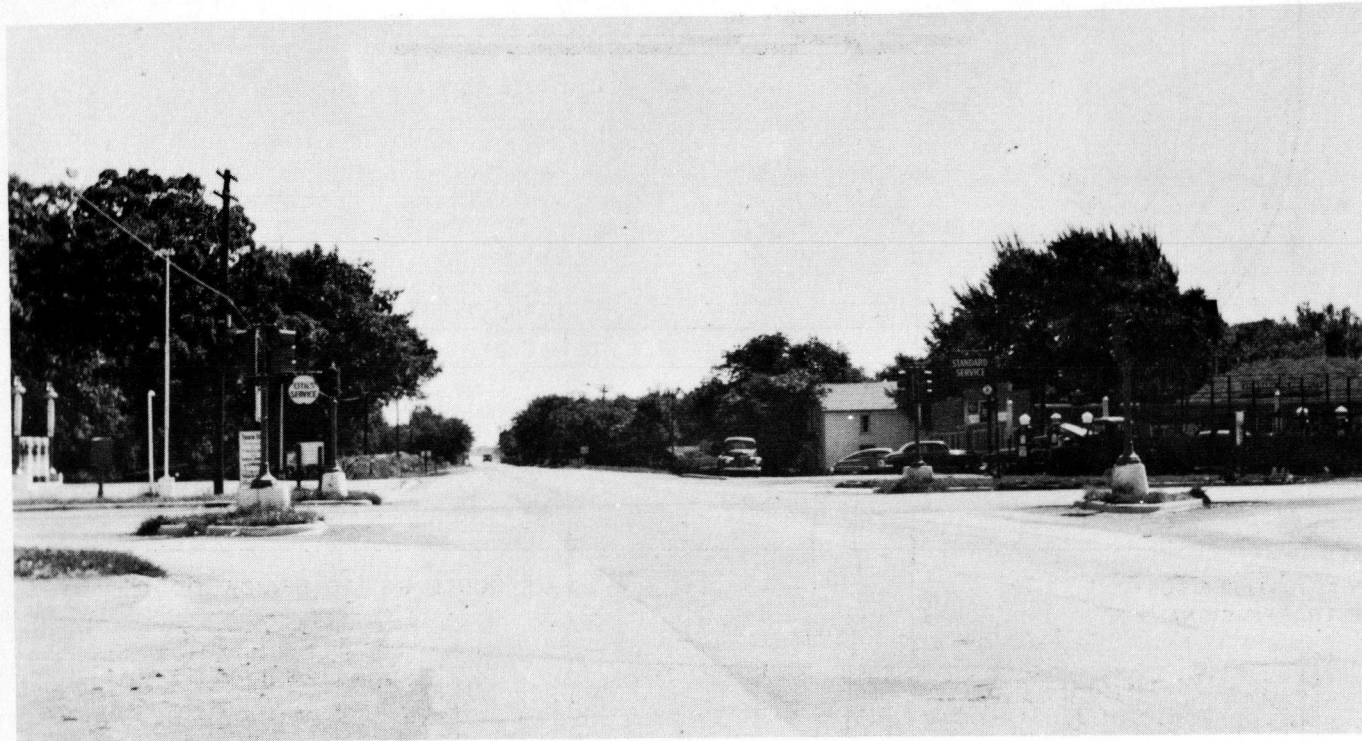
Figure 1. Channelization of 4-way right-angled intersection of US 52 and US 66, Illinois District 1.
