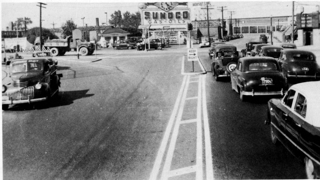
Figure 1. View of intersection of Northern Artery and Mystic Cross Avenue, Somerville, Massachusetts, after channelization showing median and triangular islands added to channelize open area at a four-way crossing under traffic-signal control.
