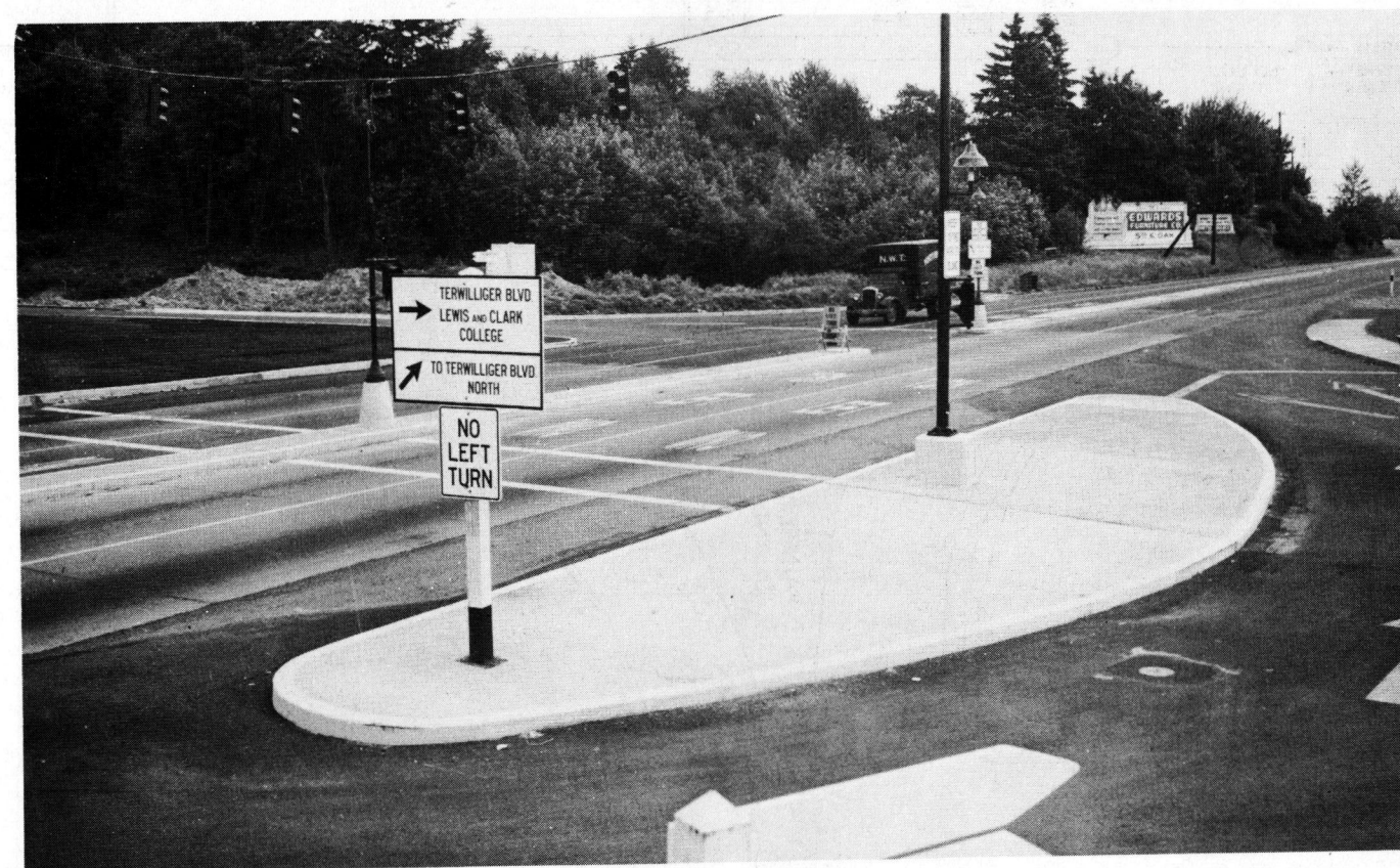
Figure 3. Details of channelizing island and traffic-control devices.
