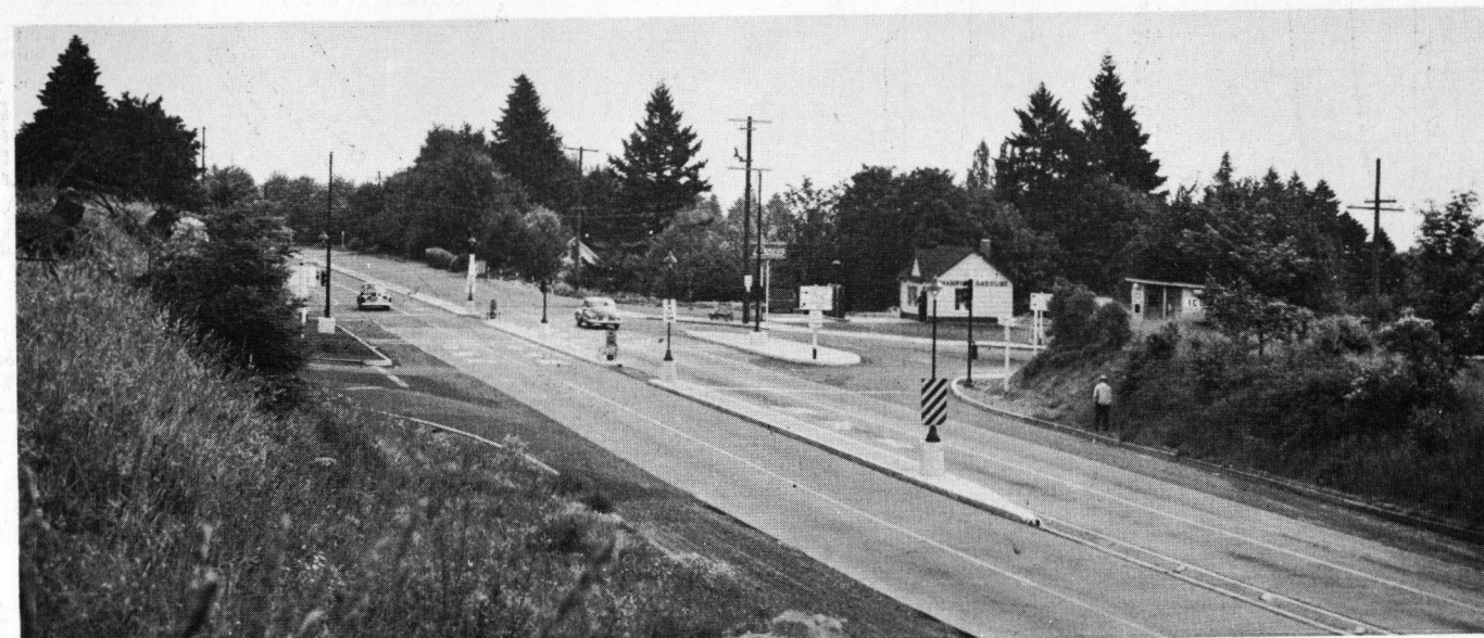
Figure 2. Split-circle treatment of main and secondary highway in which through traffic continues directly and left turns from main highway and cross traffic are deflected to right around islands. Satisfactory results are reported.
