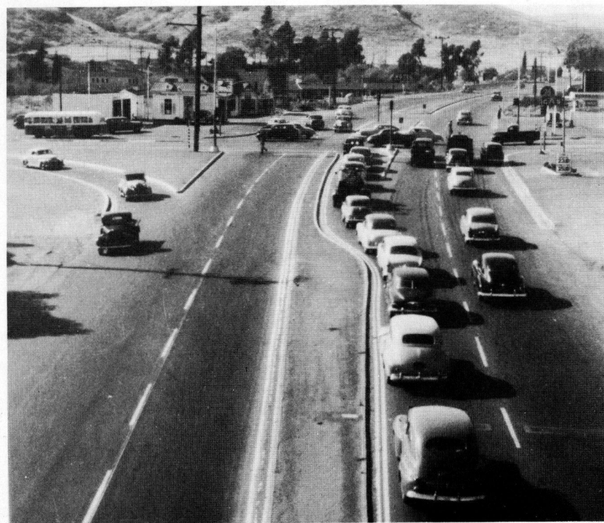
Figure 2. Intersection after channelization with details of separated left-turn lane.
