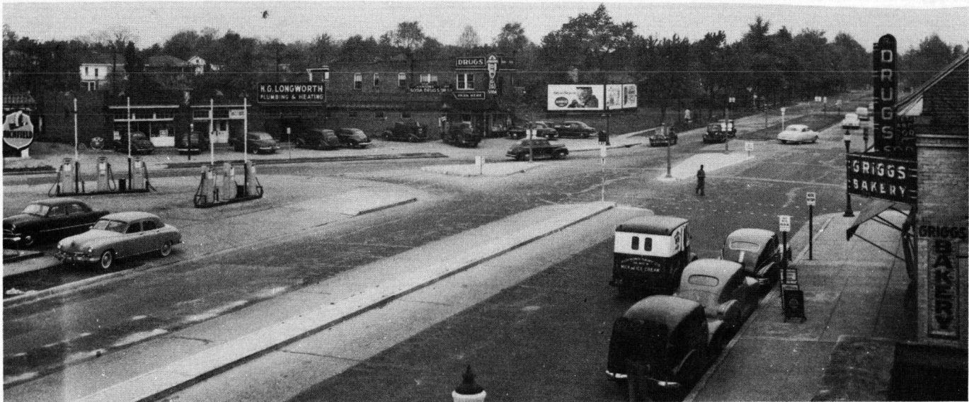
Figure 1. Channelized intersection of Chamberlayne Avenue (US 1), Lombardy Street, and Lancaster Road in Richmond, Virginia.
