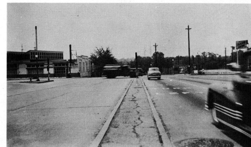
Figure 3. Looking south of Goodfellow Boulevard. The small island at the left has been used for locating a traffic-control signal, street-lighting standard, and fire hydrant.
