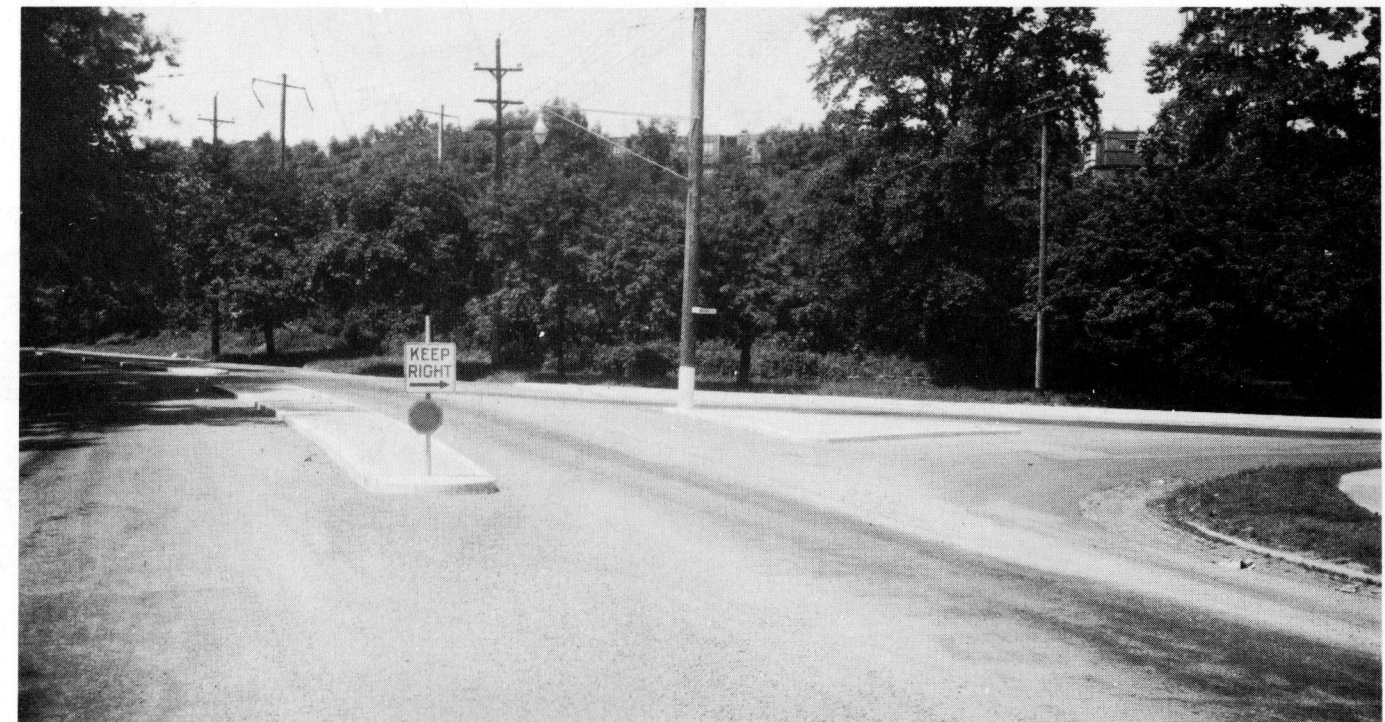
Figure 4. Good contrast is provided when concrete islands are used with asphalt pavements.
