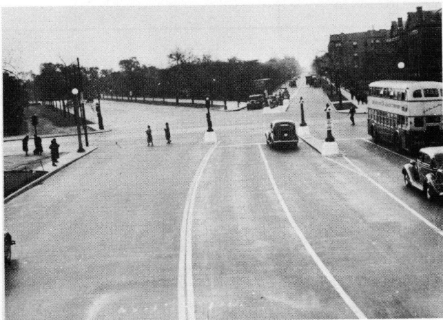
Figure 2. October 1936, after reconstruction, looking across 51st Street down South Parkway at right. Safety islands and lightposts are part of improvement.
