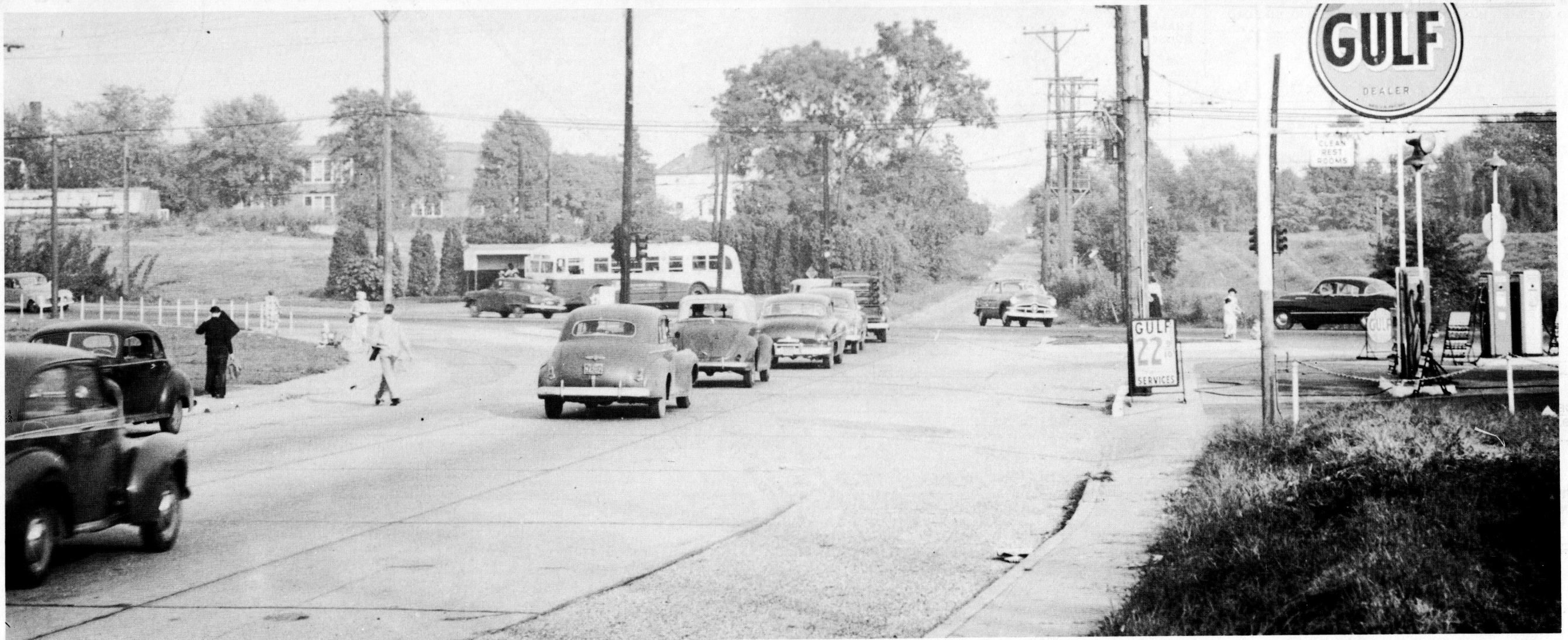
Figure 1. Channelized intersection of Maryland Avenue, Boxwood Road, and Middleborough Road. Note the pedestrian barrierfence at the left of the intersection.
