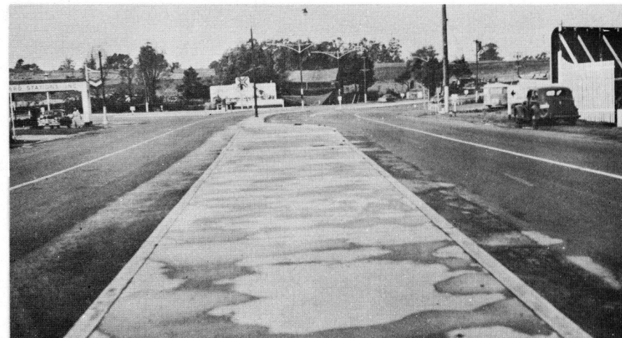
Figure 2. View of the added left-turn lane as seen from the south approach along El Camino Real.
