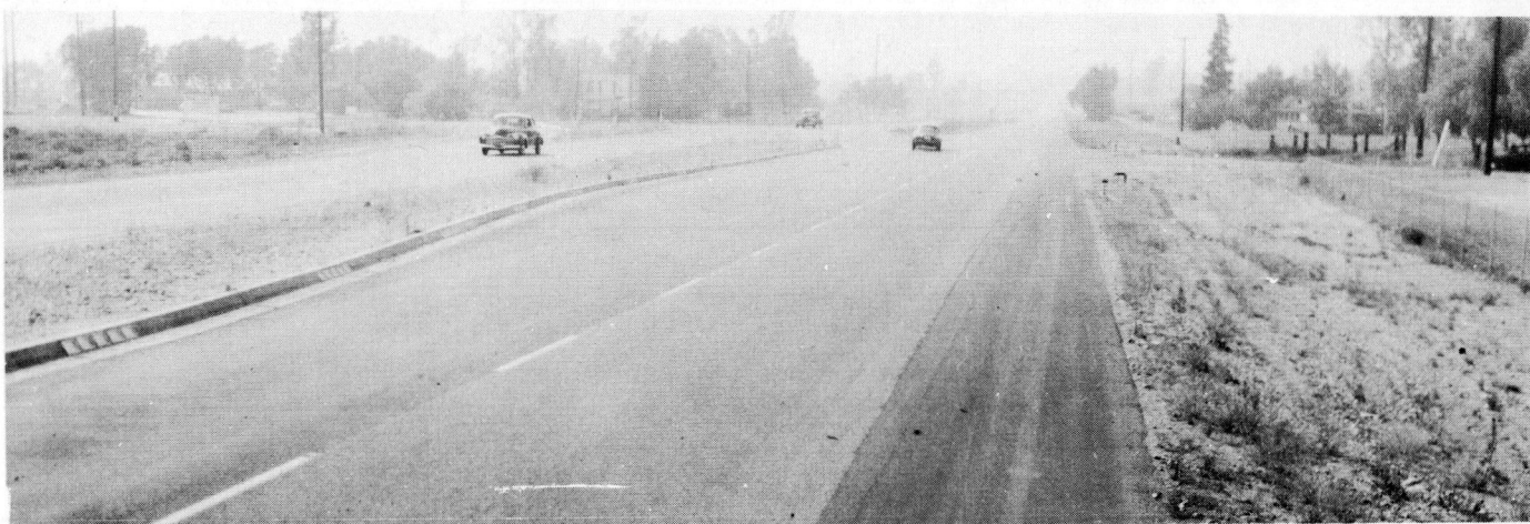
Figure 2. Looking north on US 190, showing the deceleration area and the added left-turn lane
