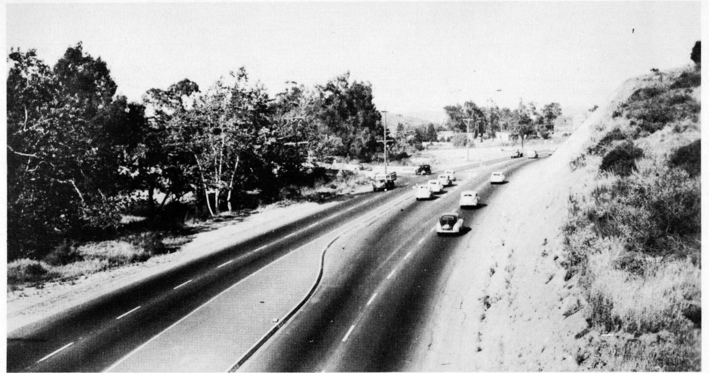
Figure 2. Intersection after channelization. Highway widened and curbed median added. Four vehicles in protected median lane, awaiting opportunity to turn left.
