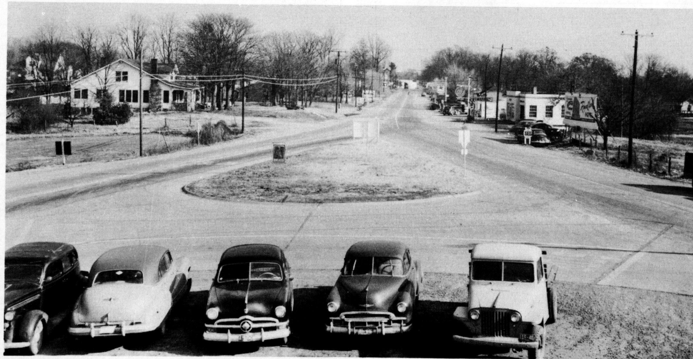
Figure 1. Channelized intersection of US 79 and US 41A, near Clarksville, Tennessee.
