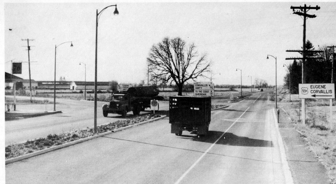
Figure 2. Looking southwest from the McMinnville leg towards Willamina. Note the modern lighting used in connection with channelization of a rural intersection.
