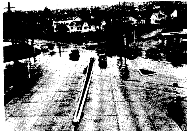
Figure 1. Channelization of multiway intersection of Green Lake Way and 50th Street Seattle. Note the pavement level beacon at the approach end of the median in the foreground.
