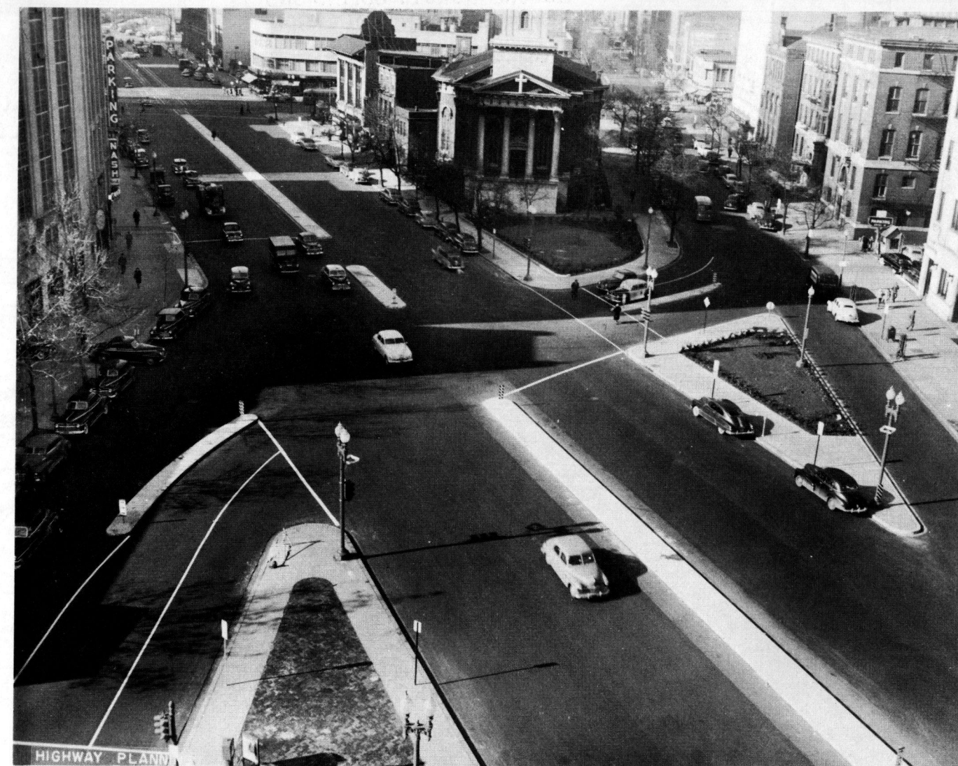
Figure 2. Completed channelization of intersection. Note the good contrast achieved between the concrete islands and the asphalt street surface.
