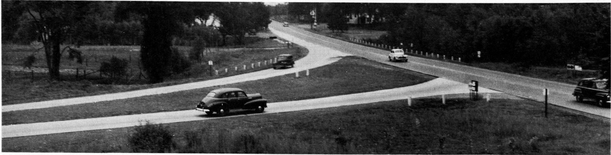
Figure 1. Channelized intersection of US 9 and Mechanicville Road (New York 236), looking south.
