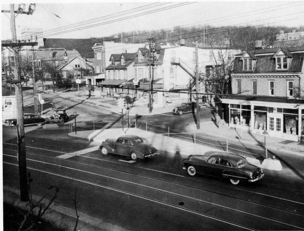
Figure 1. Channelization of the intersection of Carlisle Street, Hanover Avenue, and Hamilton Street in Allentown, Pennsylvania.
