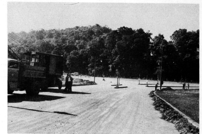
Figure 3. Elaborate channelization with multiplicity of islands requires floodlights and numerous signs to insure effective operation.
