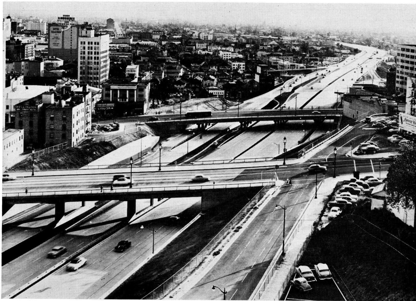
FIGURE 2 Taking land for highway construction in a heavily built-up area gives rise to many complex condemnation problems.
