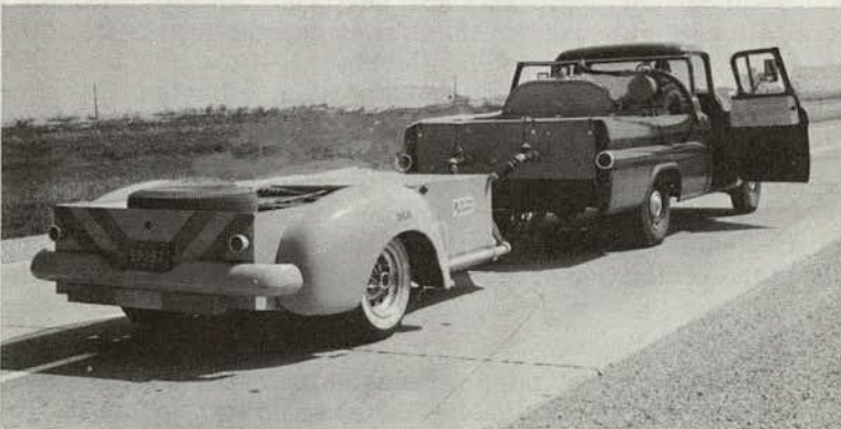
Figure 2. General Motors skid trailer.
