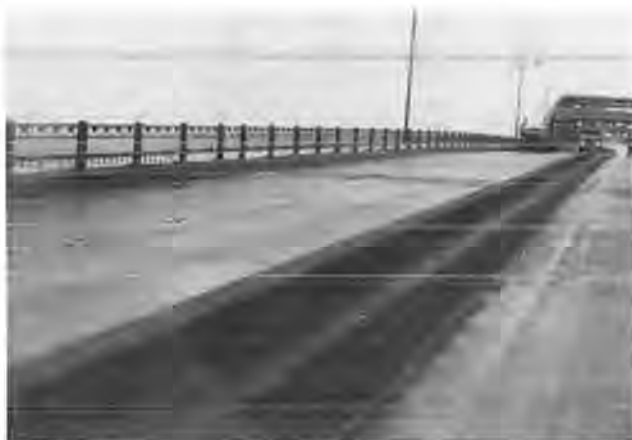
FIGURE 6 Eastbound lanes of the Calcasieu River Bridge over Lake Charles.
