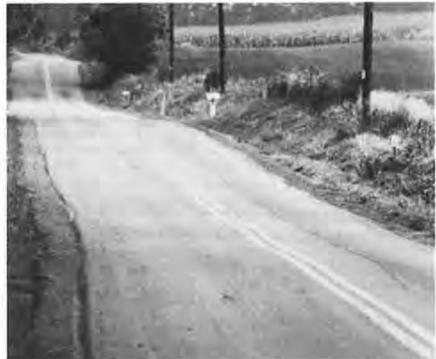
FIGURE 2 Road with washboard sections (control may be lost at speeds greater than 35 mph).
