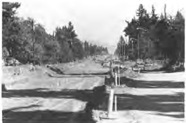
FIGURE 5 LRT construction begins after RFP landscape completed.
