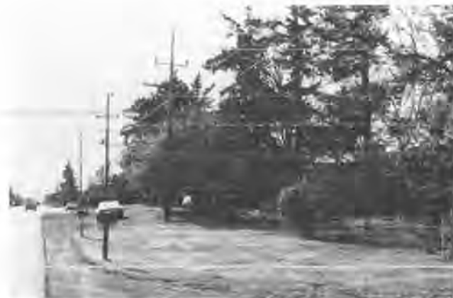
FIGURE 1 East Burnside Street before construction.
