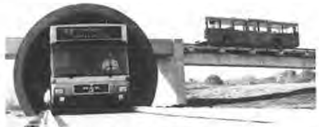
FIGURE 5 Prefabricated roadway sections.
