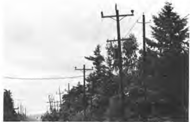
FIGURE 4 Utility poles being replaced.
