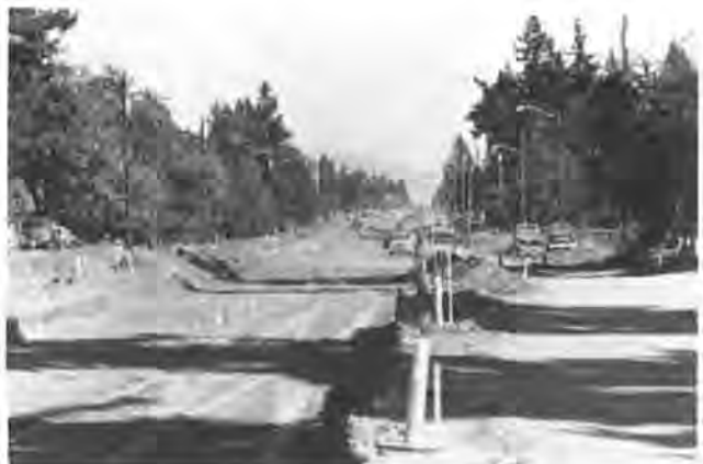
FIGURE 5 LRT construction begins after RFP landscape completed.
