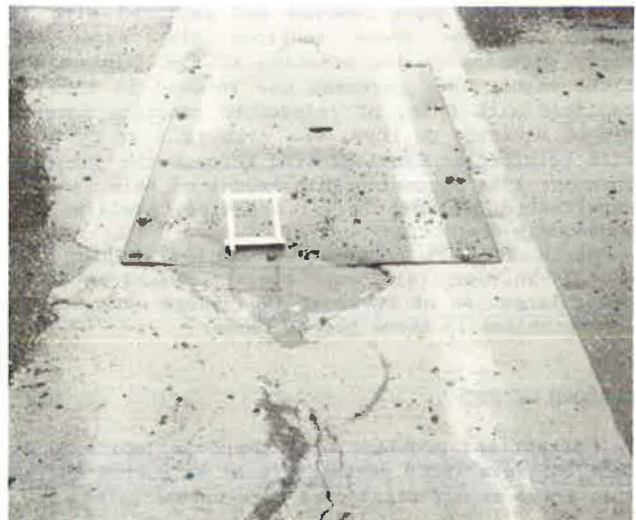
FIGURE 4 Patching of slab with metal plate.
