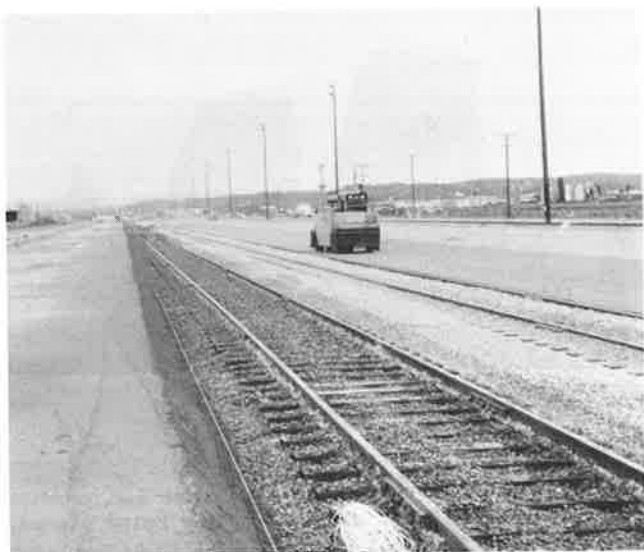
FIGURE 8 Free pavement edge at trackside loading bay.
