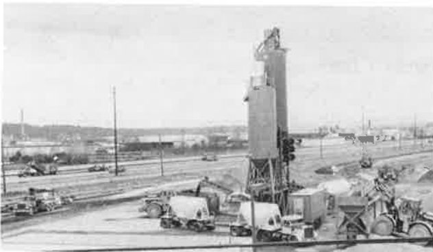
FIGURE 5 RCC batch plant.
