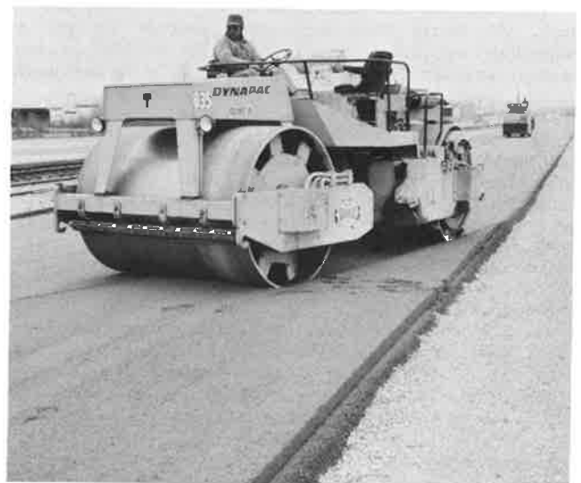
FIGURE 7 15-ton vibratory roller.
