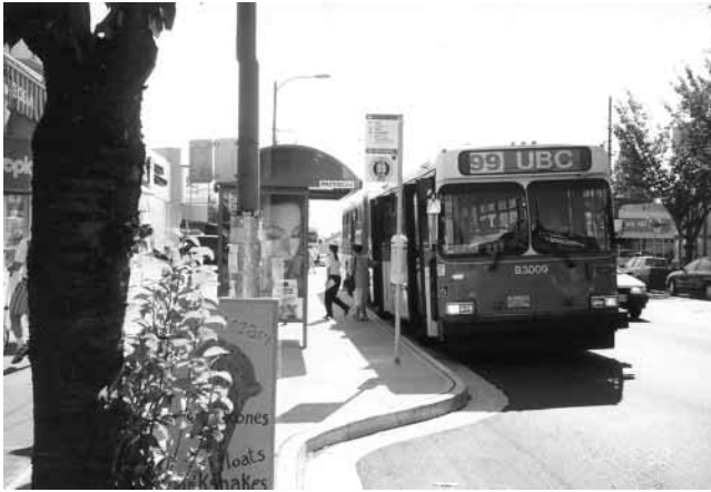
Figure A-28. Westbound bus bulge: west 10th Avenue at Sasamat Street.
