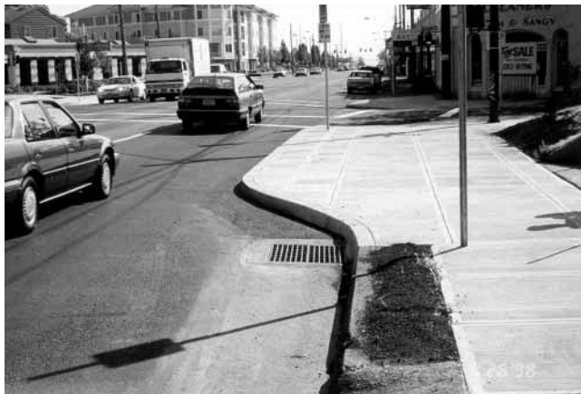
Figure A-42. Nearside bus bulb on north Sandy Boulevard at northeast 67th Avenue (looking downstream).
