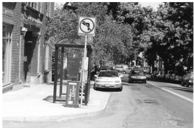
Figure A-49. Example of a narrow bulb (northwest 23rd Avenue and Burnside Street).
