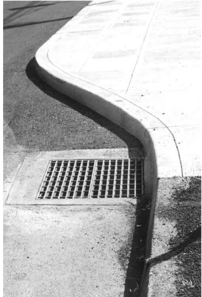
Figure A-39. Typical upstream drainage.
