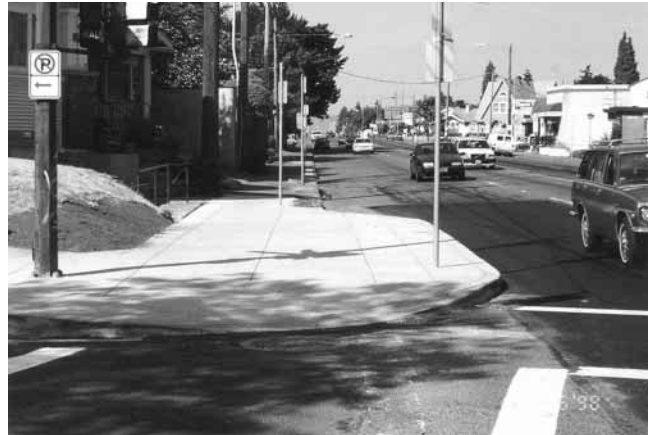
Figure A-43. Nearside bus bulb at north Sandy Boulevard at northeast 67th Avenue (looking upstream).
