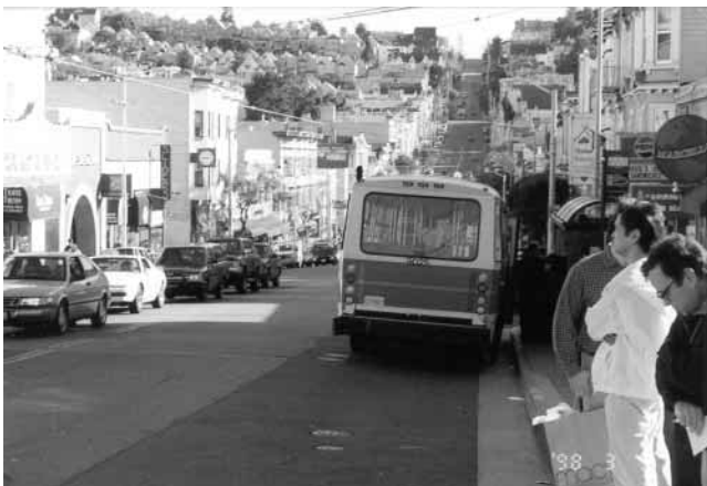
Figure A-24. Farside bus bulb on Castro Street at Market Street.
