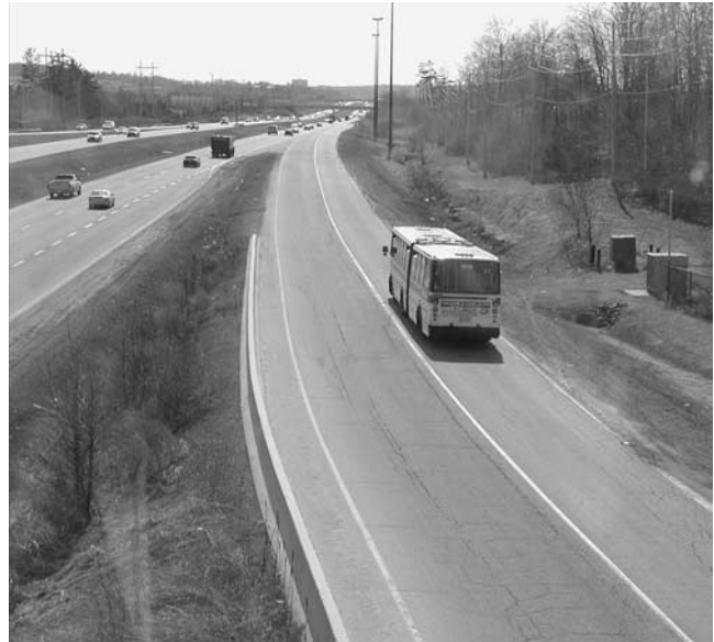
Photo 3-I. Queensway Busway shoulder lane, Ottawa.
