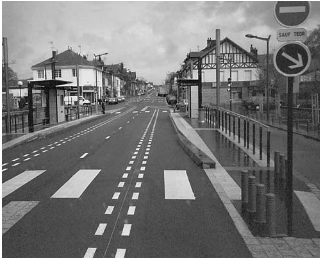
Photo 6-V. BRT running way with dashed lines for optical guidance system (Rouen, France).
