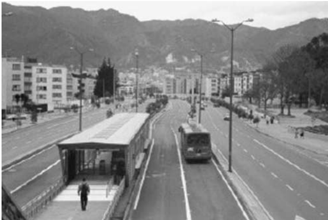
Photo 3-C. Median arterial busway, Bogotá.
