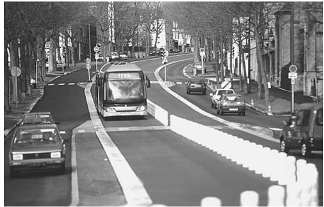
Photo 3-E. Median running way, Rouen, France, TEOR system.
