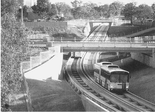
Photo 7-G. BRT guideway, Adelaide.
