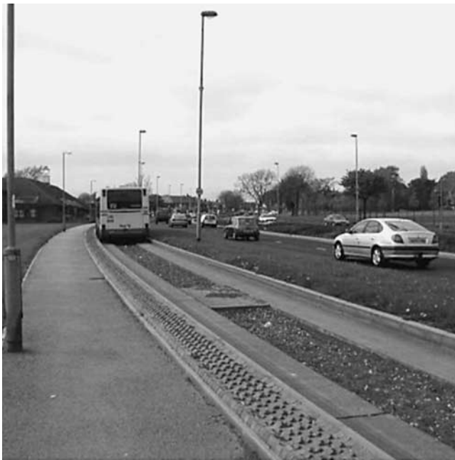
Photo 7-H. BRT guideway, Leeds.
