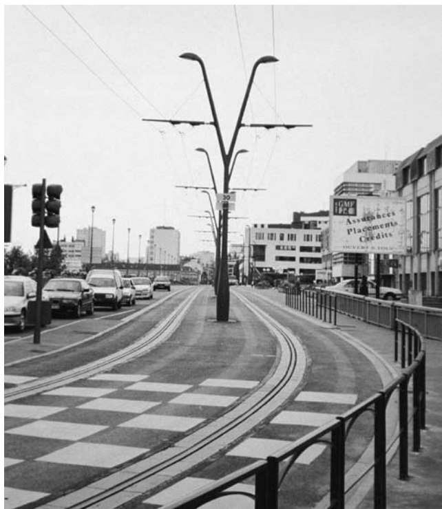
Photo 6-S. Running way incorporating guidance track used by Bombardier GLT vehicles (Nancy, France).
