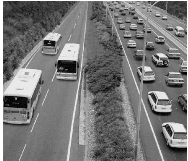
Photo 3-G. Busway adjacent to freeway, Brisbane, Australia.
