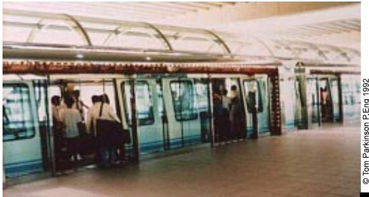
Exhibit 3-61 Orlando Airport People-Mover Doorways
