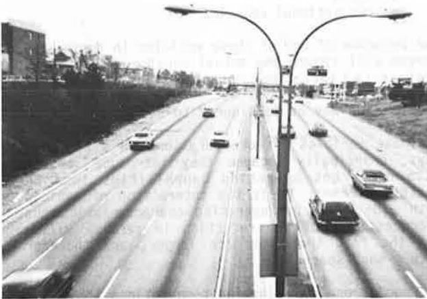
Illustration 2.3 Ideal geometric conditions are evident here. The safety-type median barrier does not pose an obstruction for capacity purposes.
