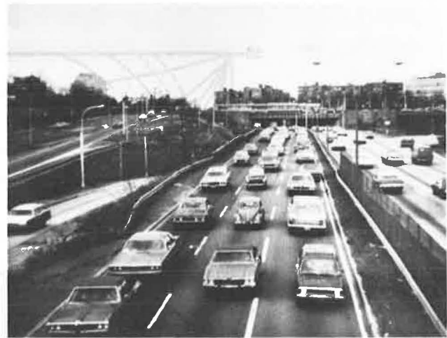
Illustration 1.4 In this case, vehicles shy away from the roadside barrier. Note that this causes a shift in the placement of vehicles in each lane. In all three lanes, vehicle placement is skewed towards the median.
