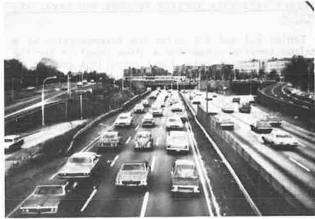
Illustration 2.2 Lateral obstructions at the roadside are 2 to 3 feet from the pavement on this freeway. The median barrier also presents an obstruction.
