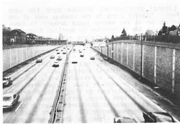
Illustration 2.4 Another freeway with ideal geometrics is shown here. The type of median barrier used does not constitute a lateral obstruction, primarily because the median lane is widened to 13 feet.
