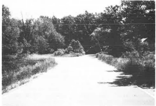
FIGURE 4: View of an intersection illustrating highway elements requiring conspicuity.
