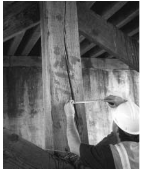
Data used to generate California Bridge Health Index involve careful measurements.
