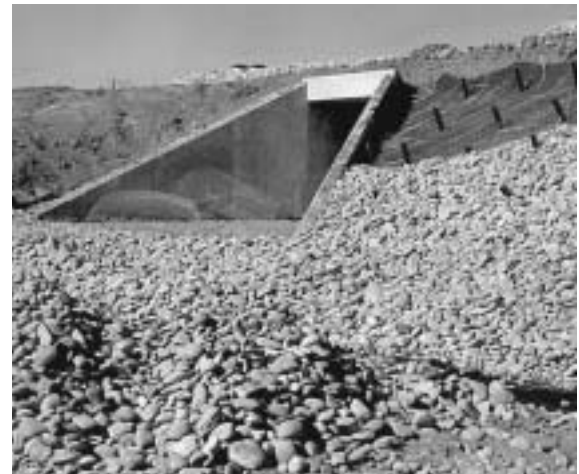
Value engineering program proposed barrier solutions on NM 44 that reduced cost but maintained quality.
