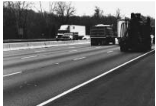
After 7 years of service with the top 4 inches of surface replaced, New Jersey I-287 remains in good condition today.
