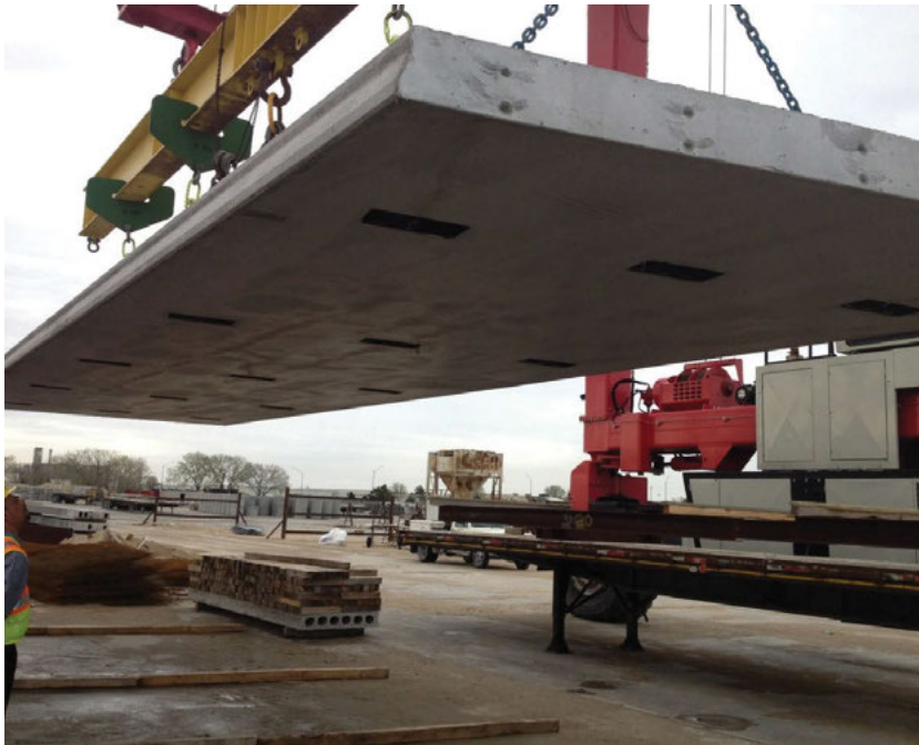
Skewed precast concrete deck panel: bottom view showing the shear pockets.
