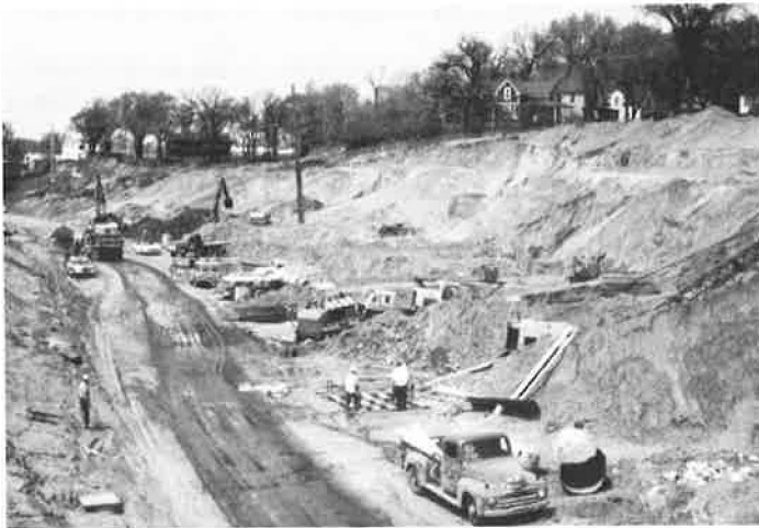
Figure 9. During construction, May 4, 1968.
