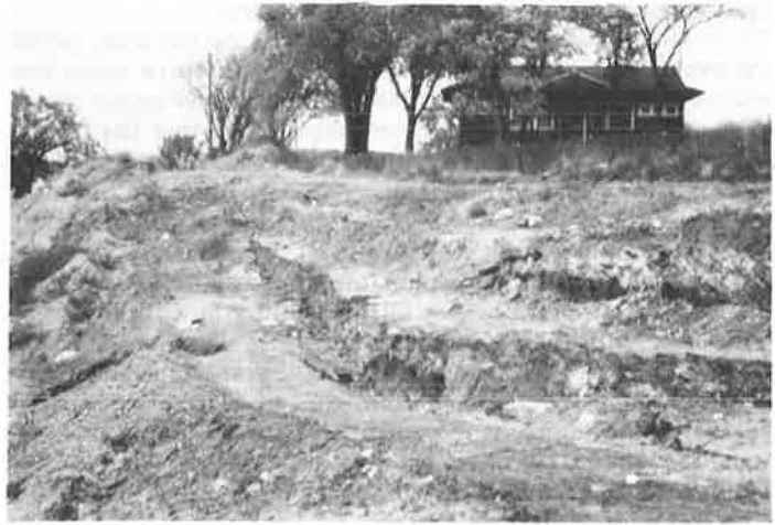
Figure 2. At Slope Indicator no. 4 looking toward railroad bridge and park.
