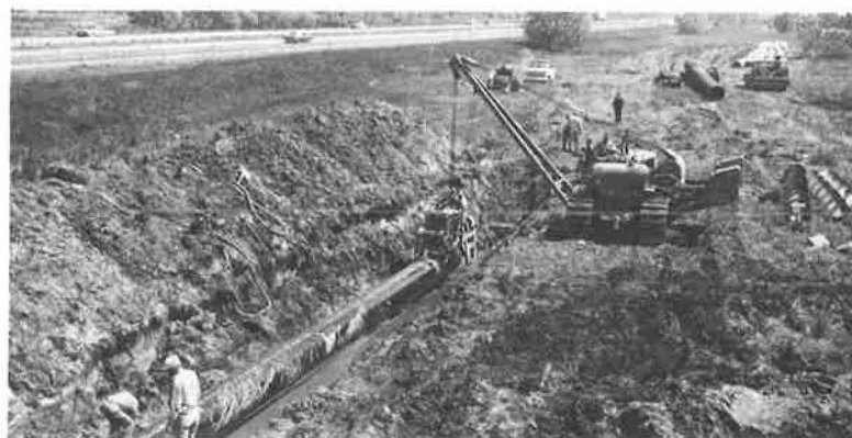
Figure 3. Road-boring equipment in operation.
