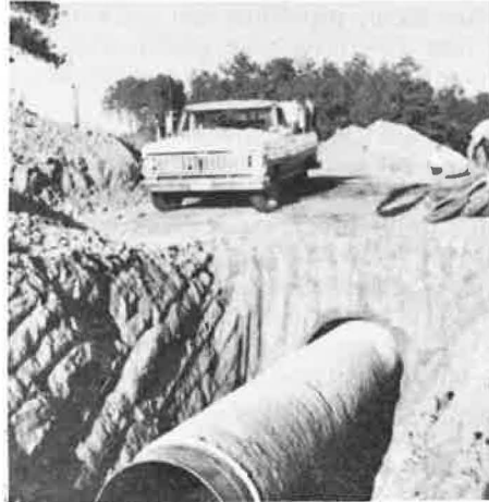
Figure 5. Uncased pipe in place before foam is applied to annular space.
