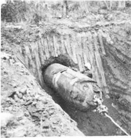
Figure 4. Pulling head being tack-welded to pipe for positioning of pipe.
