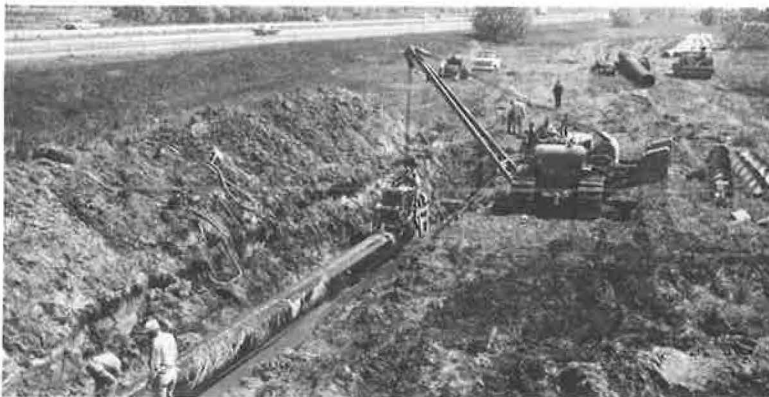
Figure 3. Road-boring equipment in operation.
