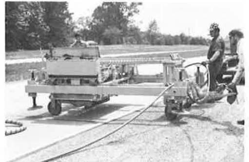
Figure 5. Klarcrete machine being turned and positioned.
