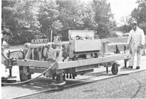
Figure 2. Klarcrete machine being positioned for operation.
