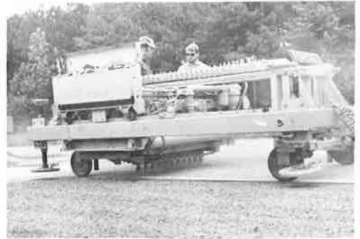
Figure 3. Klarcrete machine in operation.
