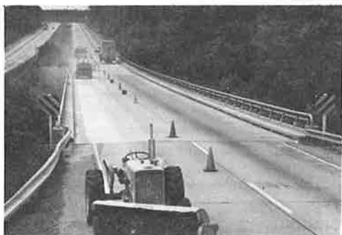
Figure 21. Long-range view of Klarcrete machine in operation on bridge deck.
