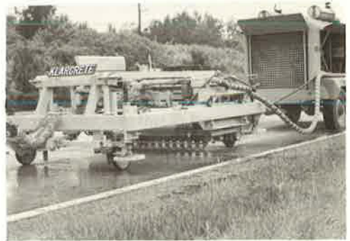
Figure 8. Klarcrete machine operating on wet pavement.
