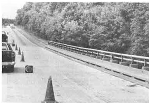
Figure 22. The southbound bridge after cleaning.
