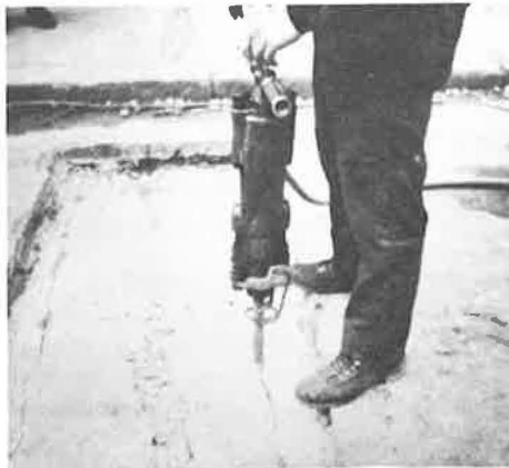
Figure 9. Use of an air hammer to break away microwave-fractured concrete.
