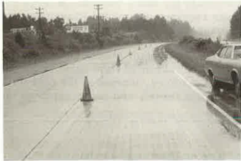
Figure 9. Wet pavement after treatment with Klarcrete machine. Note the ponding of water on the untreated portion.
