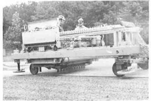
Figure 3. Klarcrete machine in operation.
