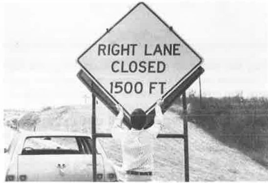
Figure 1. Research personnel positioning new signs over contractor's signs.
