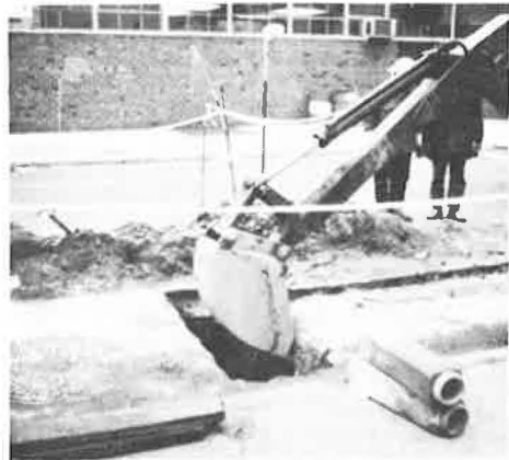
Figure 8. Backhoe removal of microwave-cracked concrete from a free edge.
