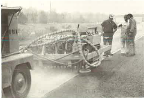
Figure 7. Dust produced by Klarcrete machine operating on dry pavement.
