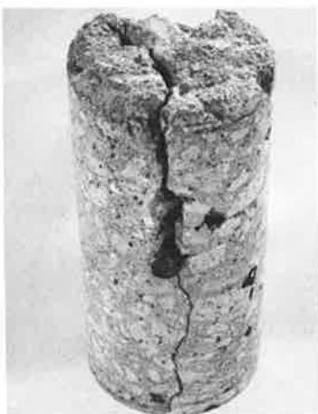
Figure 9. Core taken from a poorly consolidated pavement.
