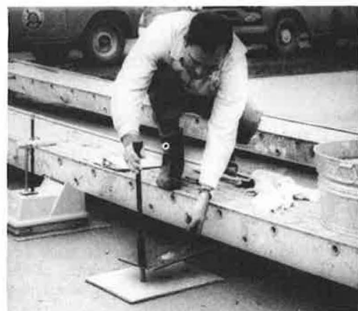
Figure 6. Taking nuclear density measurements on plastic concrete.
