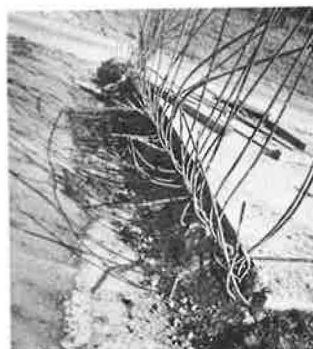
Figure 2. End arrangement of CRCP.
