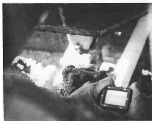
Figure 5. Using tachometer to set vibrator frequency.
