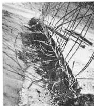
Figure 2. End arrangement of CRCP.
