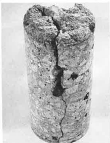
Figure 9. Core taken from a poorly consolidated pavement.
