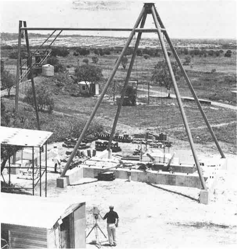
Figure 8. Southwest Research Institute pendulum impact tester.
