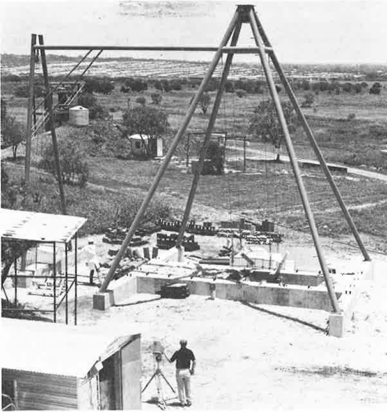
Figure 8. Southwest Research Institute pendulum impact tester.
