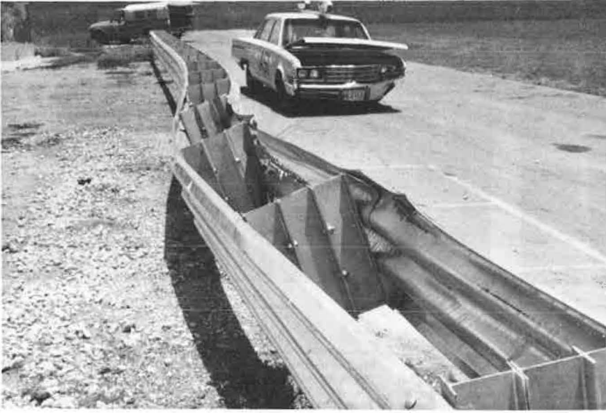
Figure 11. Beam and vehicle damage after test AS-1.
