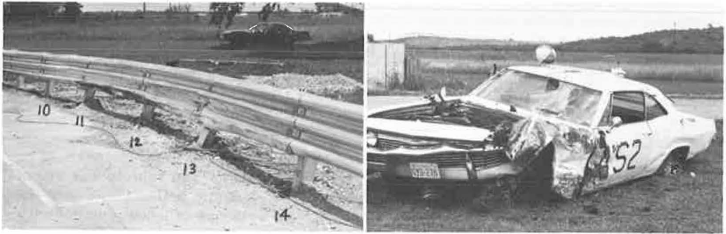
Figure 13. Beam and vehicle damage after test AS-2.
