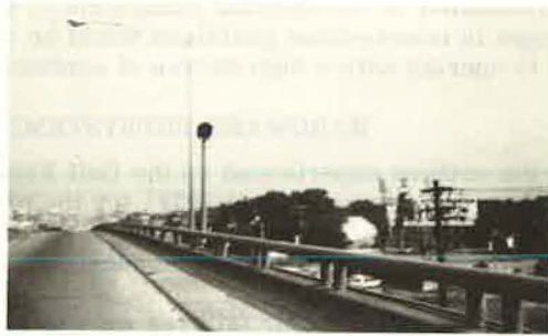
Figure 2. Flasher unit at crest of overpass.
