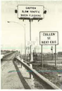
Figure 1. Warning sign with flashers.
