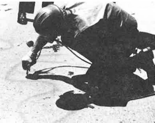
Figure 4. Injecting epoxy into undersurface structure.
