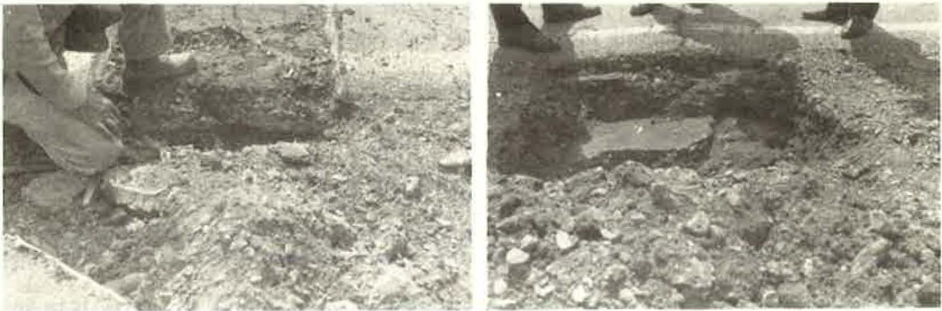
Figure 1. Two-layer soil cement failure.
