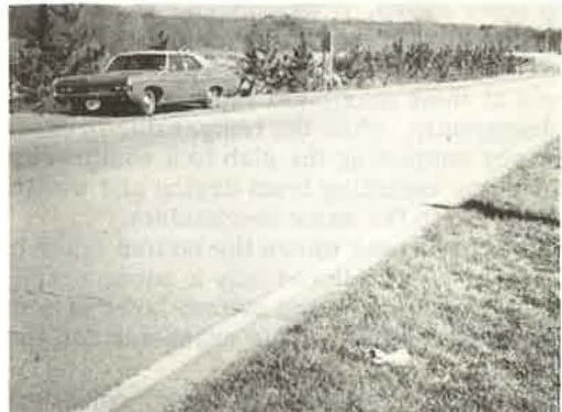
Figure 15. Pavement surface of two-layer section.
