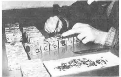
Figure 23. Fastening measuring marks to specimens.
