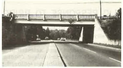
Figure 2. Park Street bridge.
